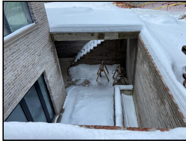
Below grade void next to proposed covered porch taken on February 24, 2025
