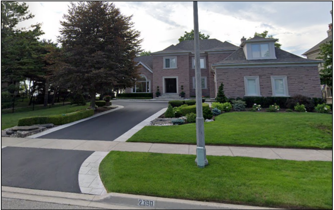
Primary Façade – 2390 Carrington Place
