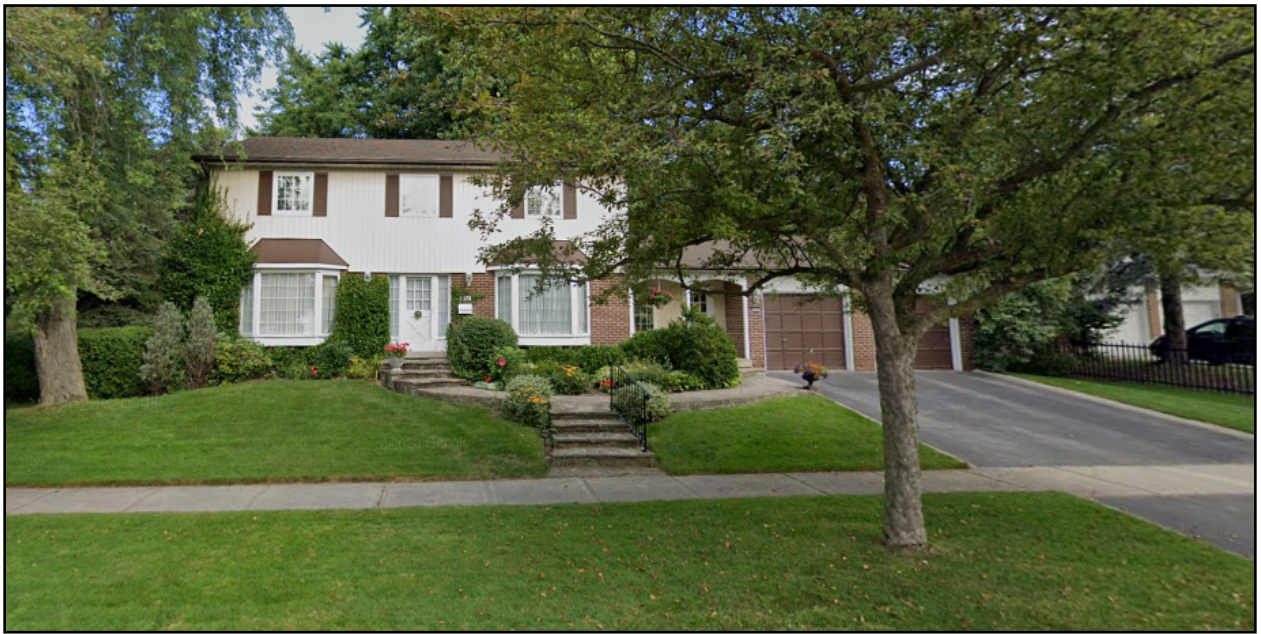
Primary Façade – 2351 Carrington Place
