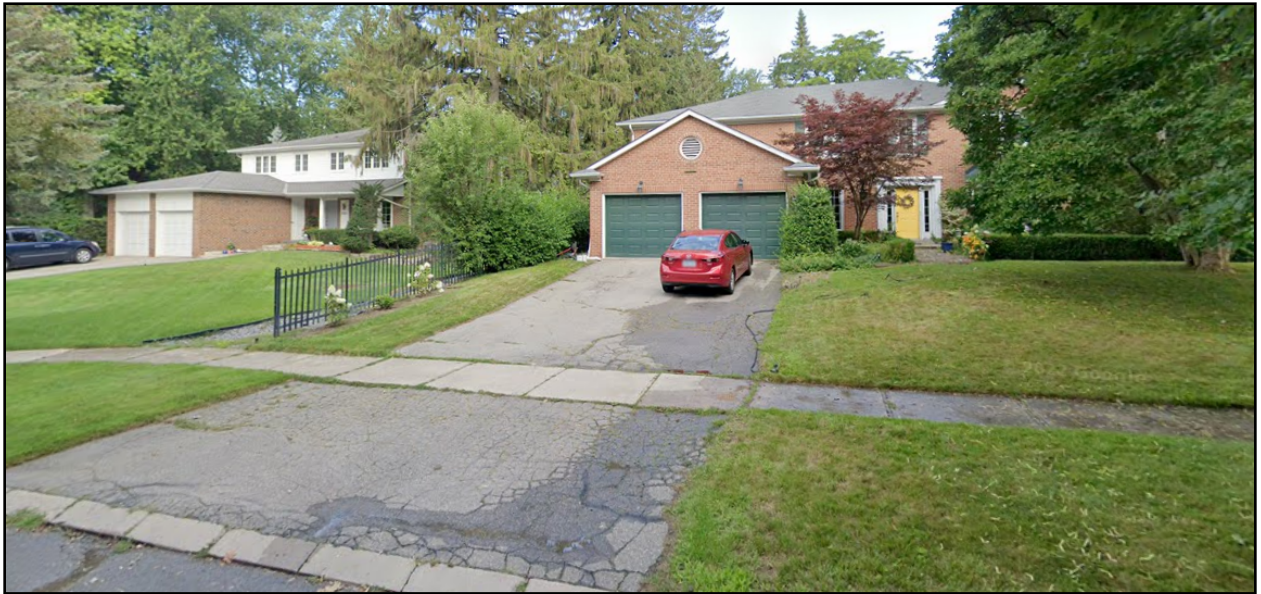
Primary Façade – 2361 & 2367 Carrington Place
