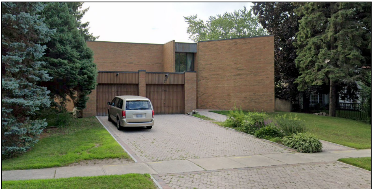
Primary Façade – 2360 Carrington Place
