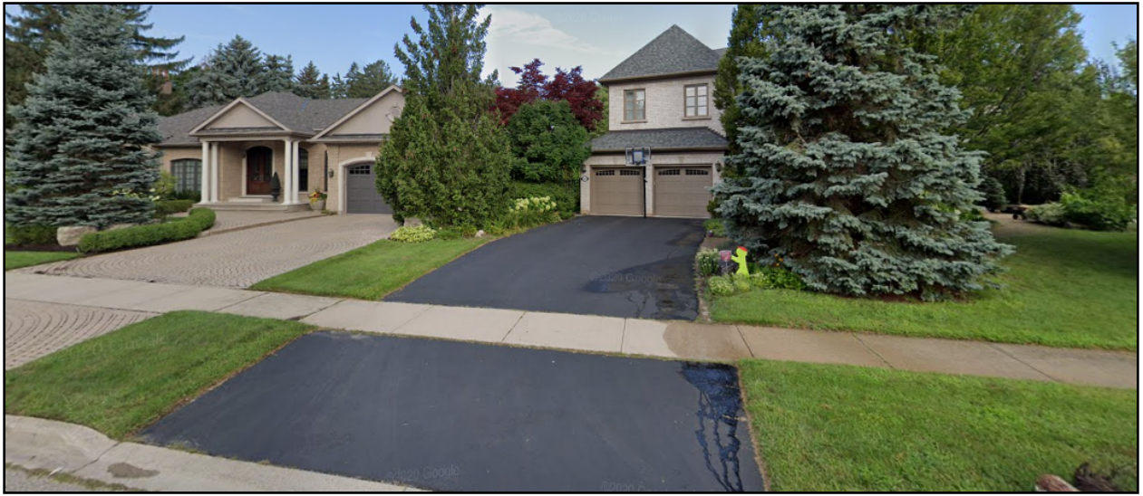
Primary Façade – 2387 & 2395 Carrington Place
