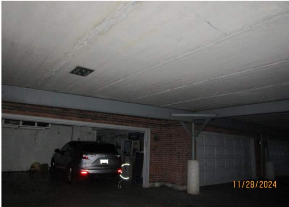
PHOTO 1: STEEL BEAM AND HOLLOW CORE SLAB
