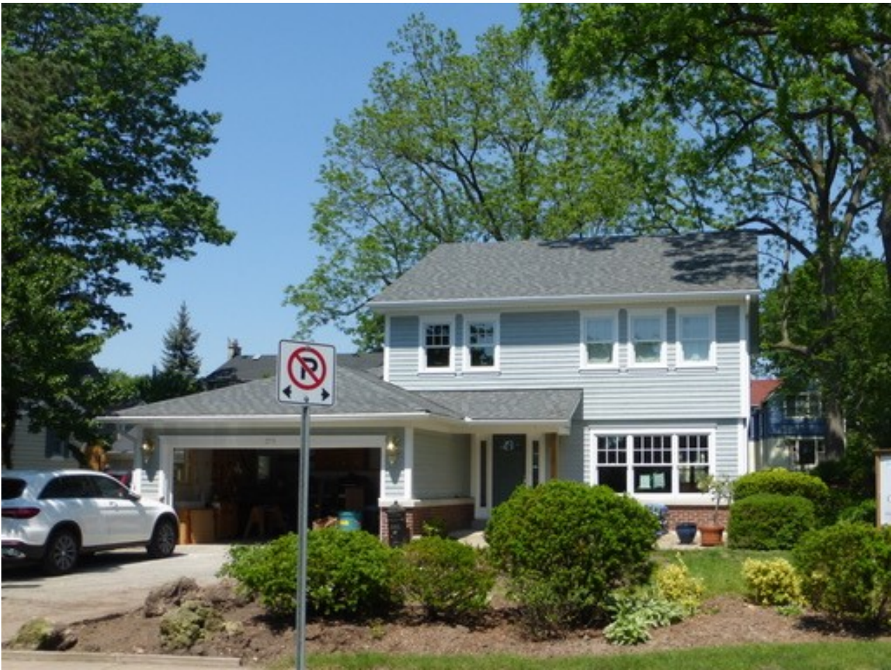
Immediately on completion of renovation in 2017.
