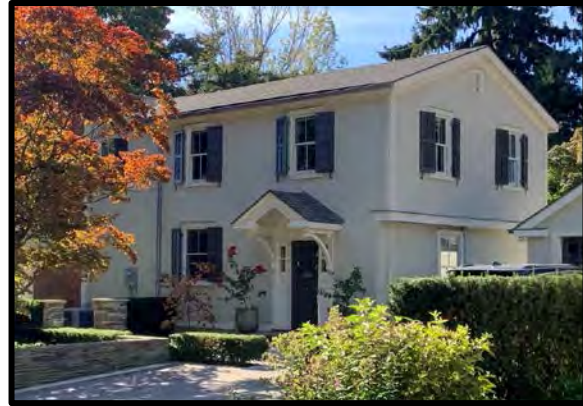
Figure 46: 53 Thomas Street (left) – Example of stucco cladding Figure 47: 22 Reynolds Street (right) – Example of stucco cladding
