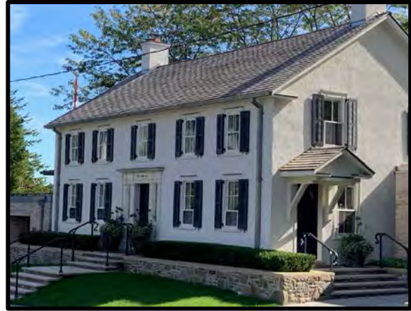
Figure 8: 212 Front Street (left) – Cedar shake hip roof with dormers and stucco cladding Figure 9: 176 Front Street (right) – Cedar shake gable roof with stucco cladding
