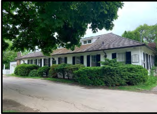
Figure 8: 212 Front Street (left) – Cedar shake hip roof with dormers and stucco cladding Figure 9: 176 Front Street (right) – Cedar shake gable roof with stucco cladding
