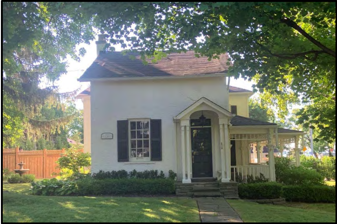
Figure 24: 212 King Street – Main entrance wood door facing street
