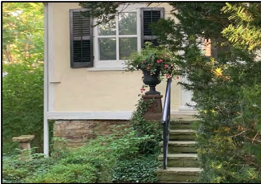
Figure 26: 115 William Street – Lakestone foundation
