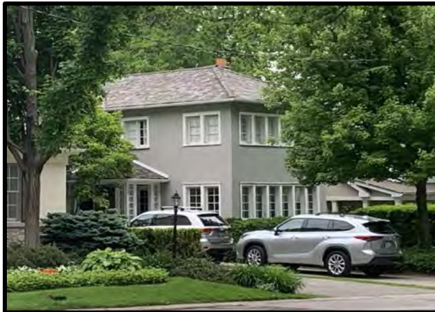
Figure 10: 329 William Street (left) – Cedar shake hip roof with stucco cladding Figure 11: 307 William Street (right) – Asphalt hip roof with horizontal wood cladding
