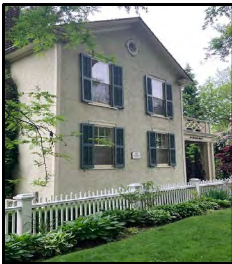
Figure 48: 29 Thomas Street (left) – Example of stucco cladding Figure 49: 19 Navy Street (right) – Example of early brick cladding
