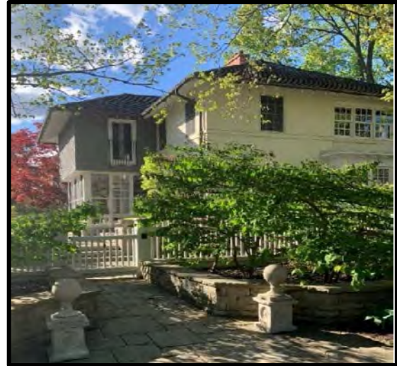
Figure 58: 273 William Street (left) – addition to west; height of addition matches; consistency in roof form and style of windows/doors and trim; complementary use of materials
