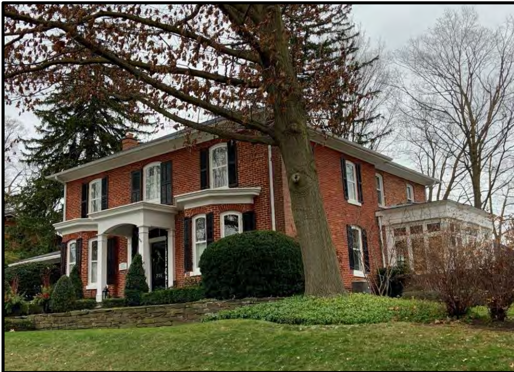
Figure 68: 226 William Street – low lying lakestone wall across front of house with soft landscaping and open vistas to westerly side yard
