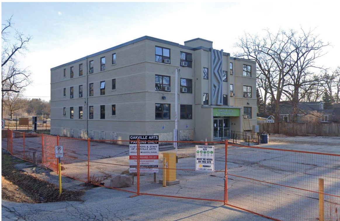
4.1.5.1.C – Existing Rear (Southwest) Elevation
