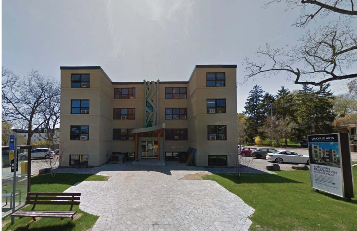
4.1.5.1.D - Existing Front (Northeast) Elevation – 2015
