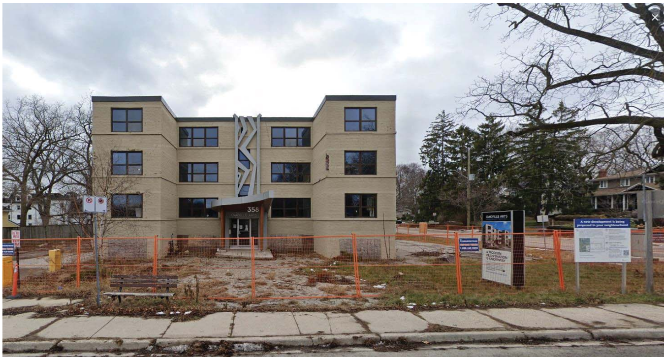
4.1.5.1.A - Existing Northeast (Front) Elevation
