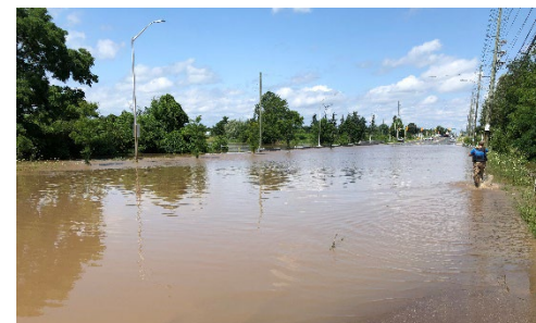
Roadway Flooding – Steeles Avenue at 6 th Line – July 16, 2024
