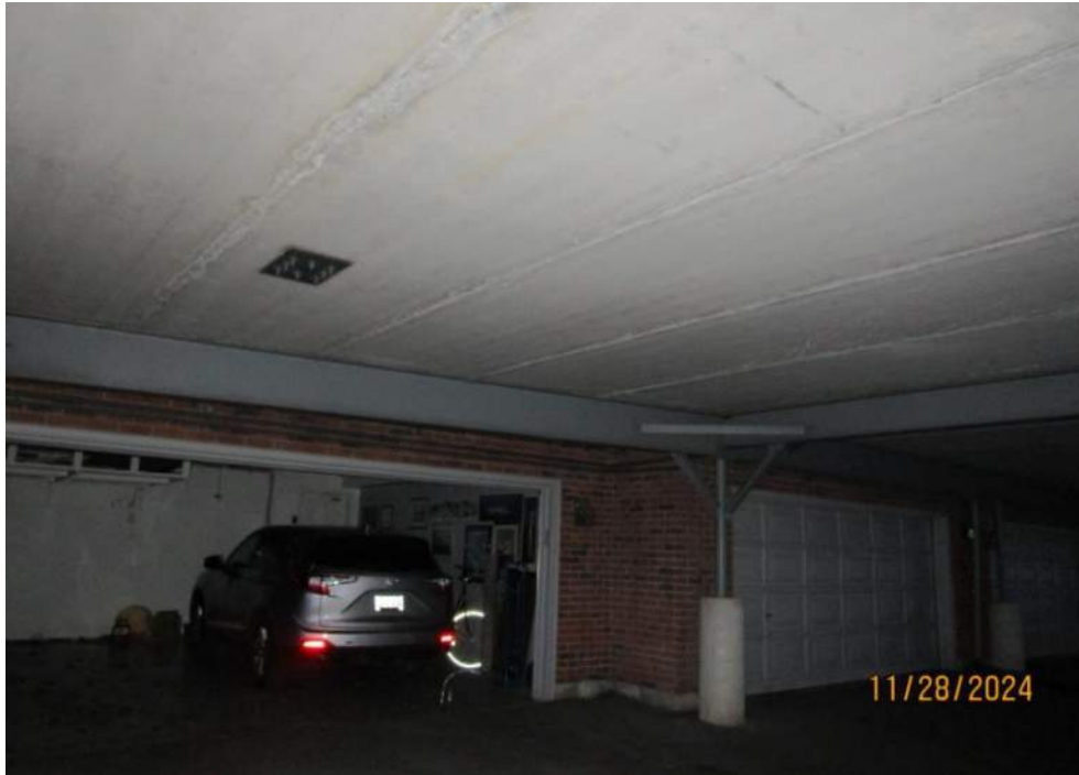
PHOTO 1: STEEL BEAM AND HOLLOW CORE SLAB
