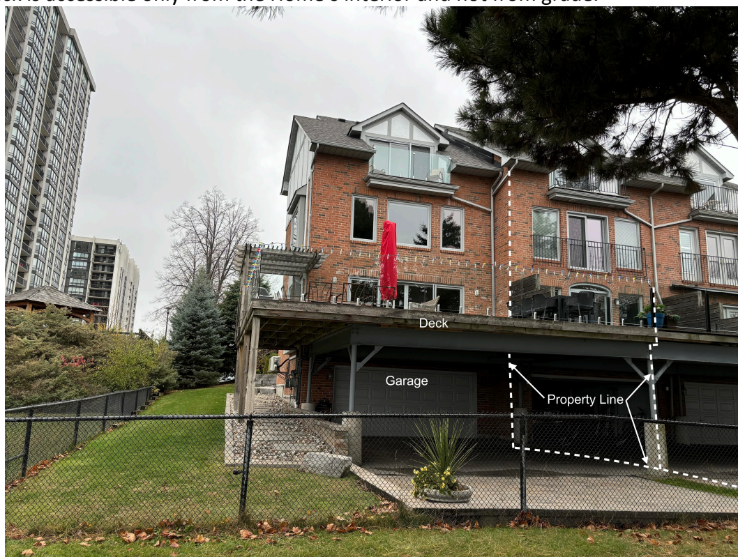
Figure 3) Photo of Existing Rear Yard Deck and Driveway access to Garage at Grade
