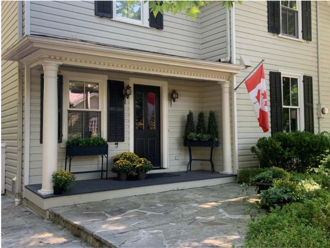
53 Dunn Street – Example of Horizontal Wood Cladding
