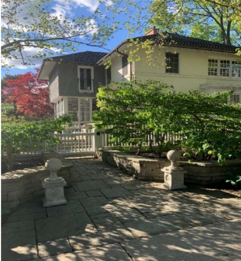
66 Dunn Street – small addition to rear and visible from side yard. Height of addition matches; consistency in roof form and style of windows/doors and trim; complementary use of materials with shake cladding distinct from stucco
