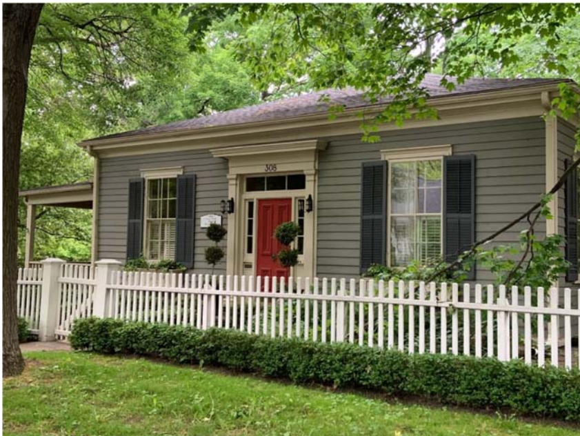
308 William Street – Wood Windows with Storm and Operating Louvered Shutters
