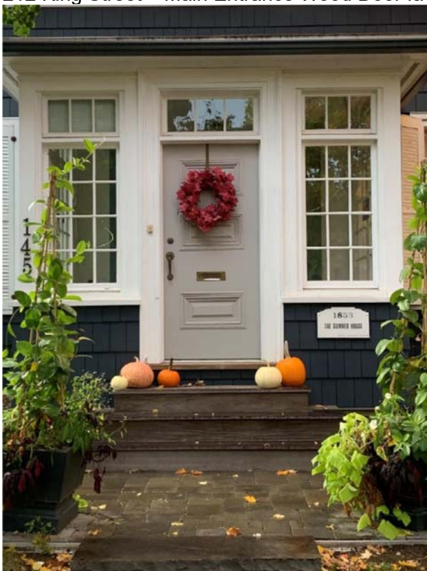
145 William Street – Main Entrance Wood Door facing street
