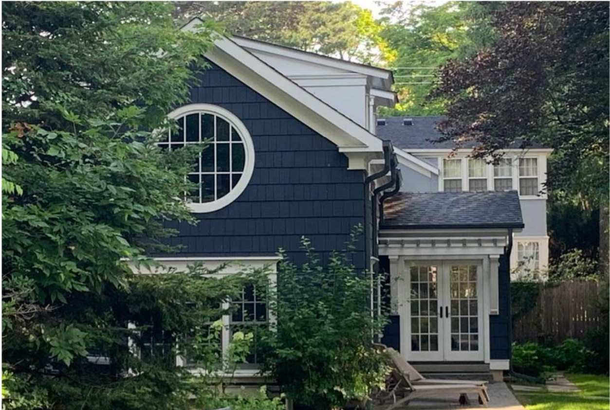
145 William Street – Separate Coach House set back in rear yard
