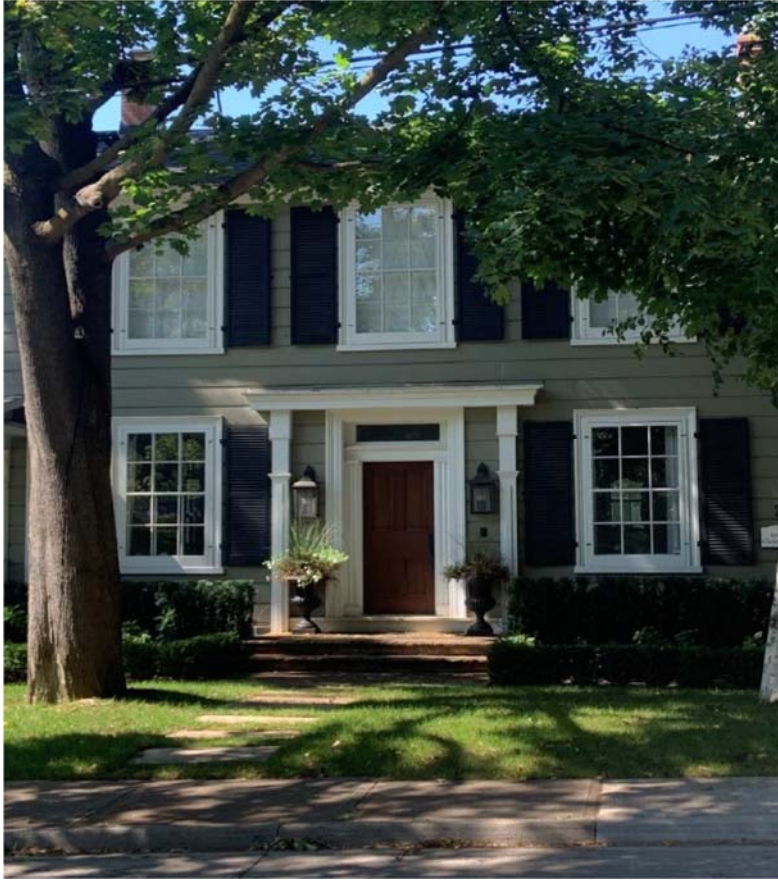
215 William Street – Wood Windows with Storm and Operating Shutters
