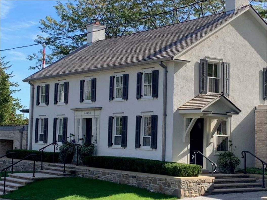
176 Front Street – Cedar Shake Gable Roof with Stucco Cladding
