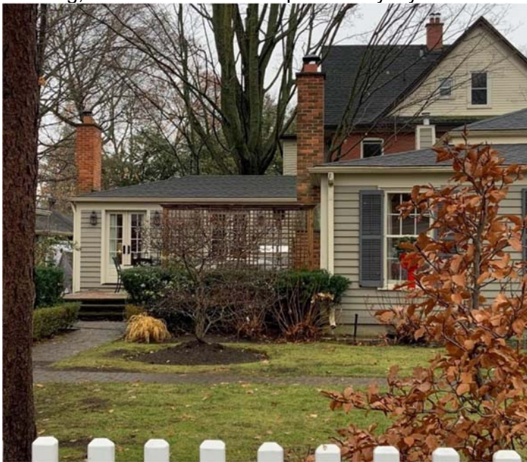
308 William Street –addition to rear and visible from Reynolds Street. Height of addition is lower than original, consistent horizontal wood cladding and chimney style, wood French doors in complementary style
