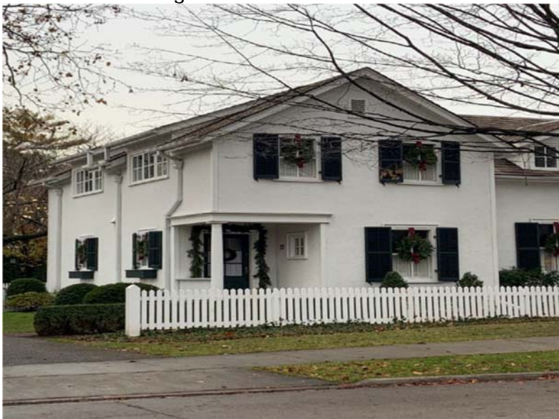
53 Navy Street – addition to rear and visible from William Street. Height of addition matches; consistency in gable roof form stucco cladding and public facing style of windows/doors and trim;
