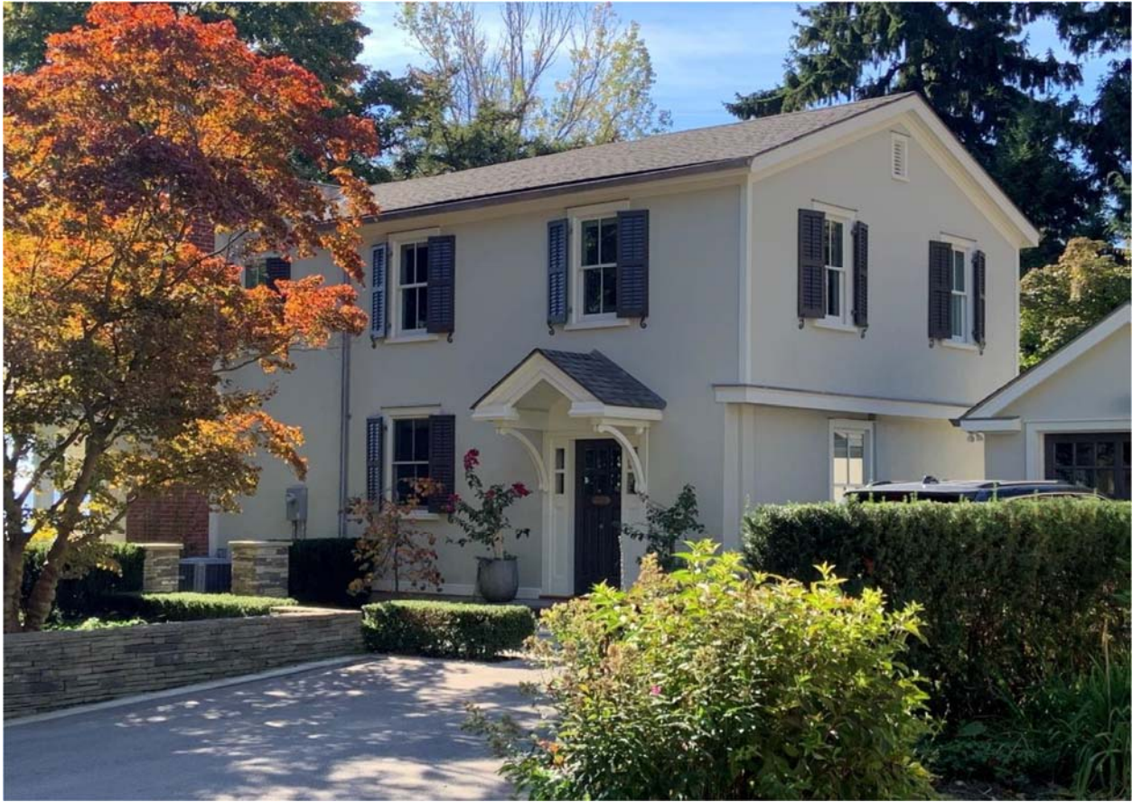
22 Reynolds Street – Example of Stucco Cladding
