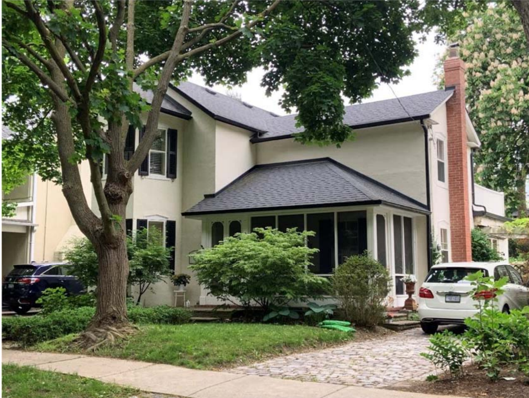
301 William Street – Asphalt Gable Roof with Stucco Cladding
