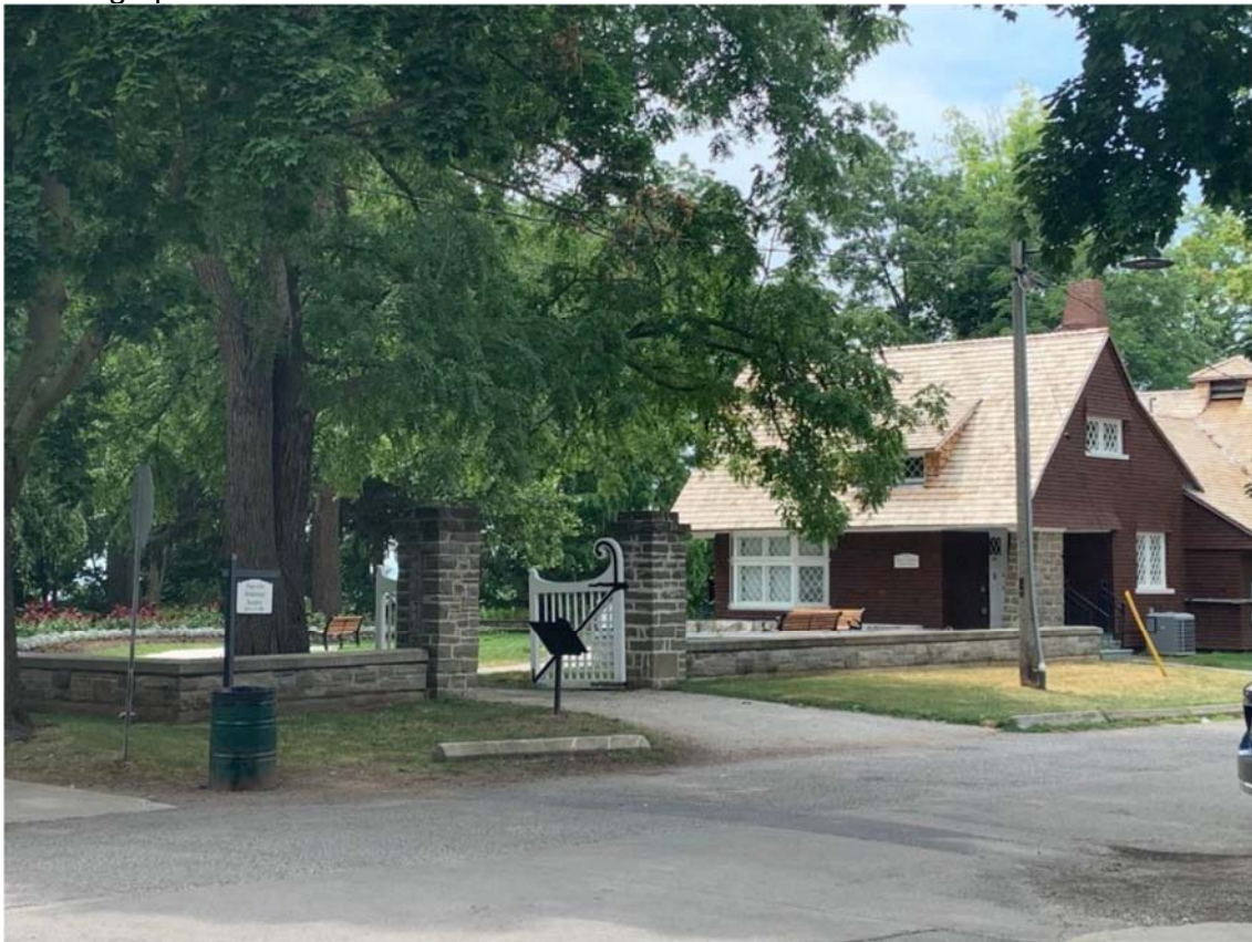
Navy Street Erchless Estate – low stone wall with stone pillars and wooden gate
