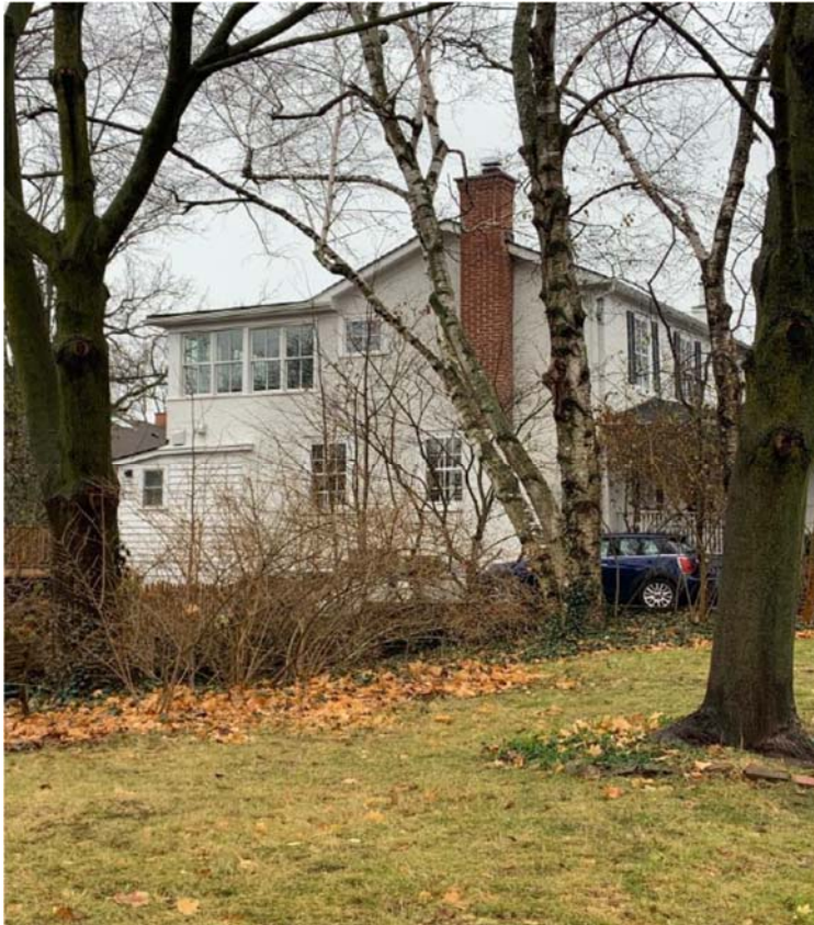
188 William Street –addition to rear and visible from William Street. Height of addition is lower than original, combination of consistent stucco cladding and complementary horizontal wood cladding; wood windows in complementary style
