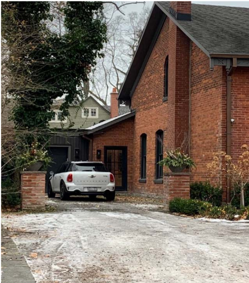
Trafalgar Road – Attached single car garage with shed appearance setback to rear of property
