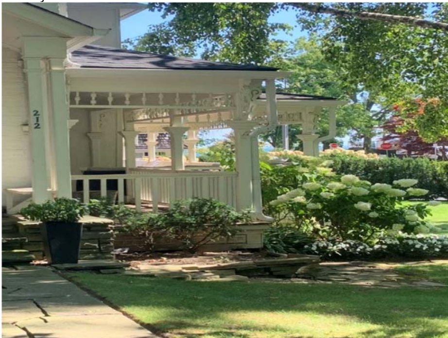
212 King Street – Covered Open Porch
