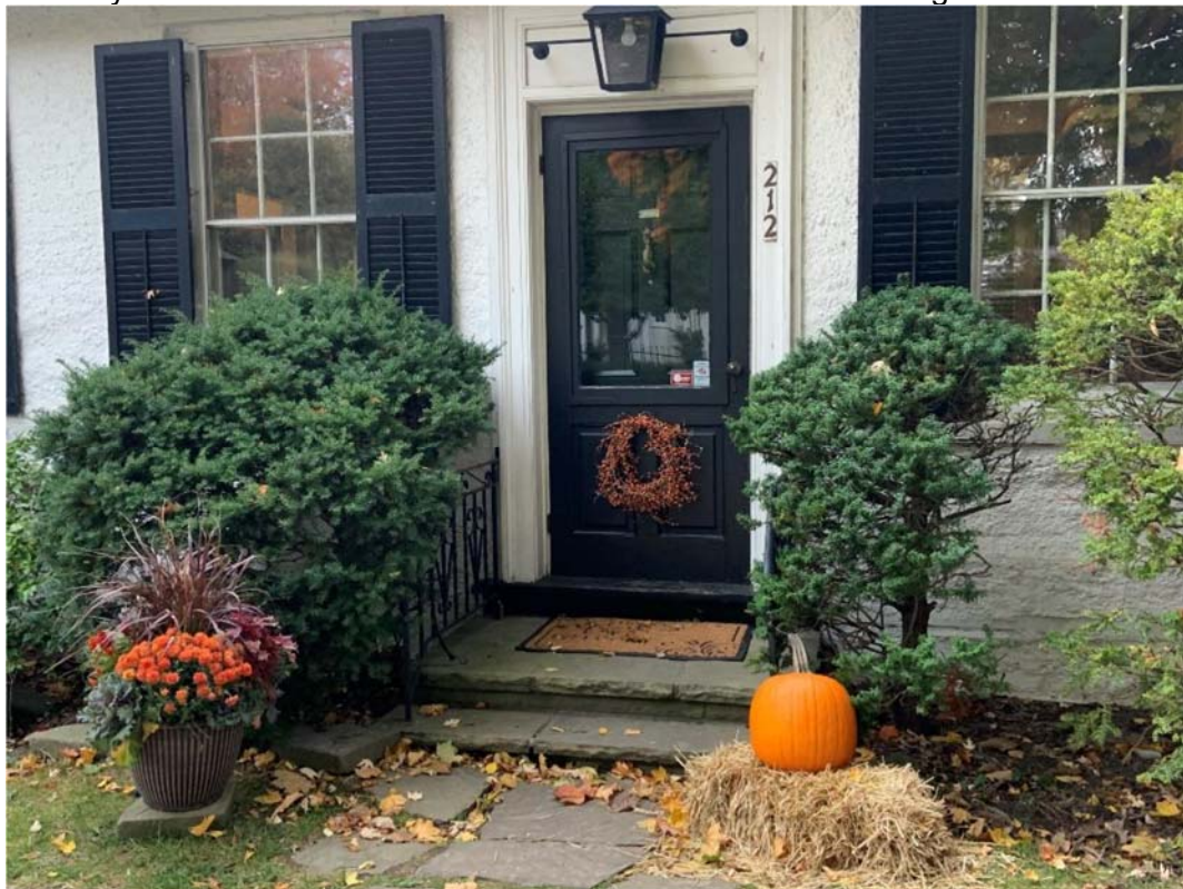
212 Front Street – Main Entrance Wood Door with Wood Storm Door facing street
