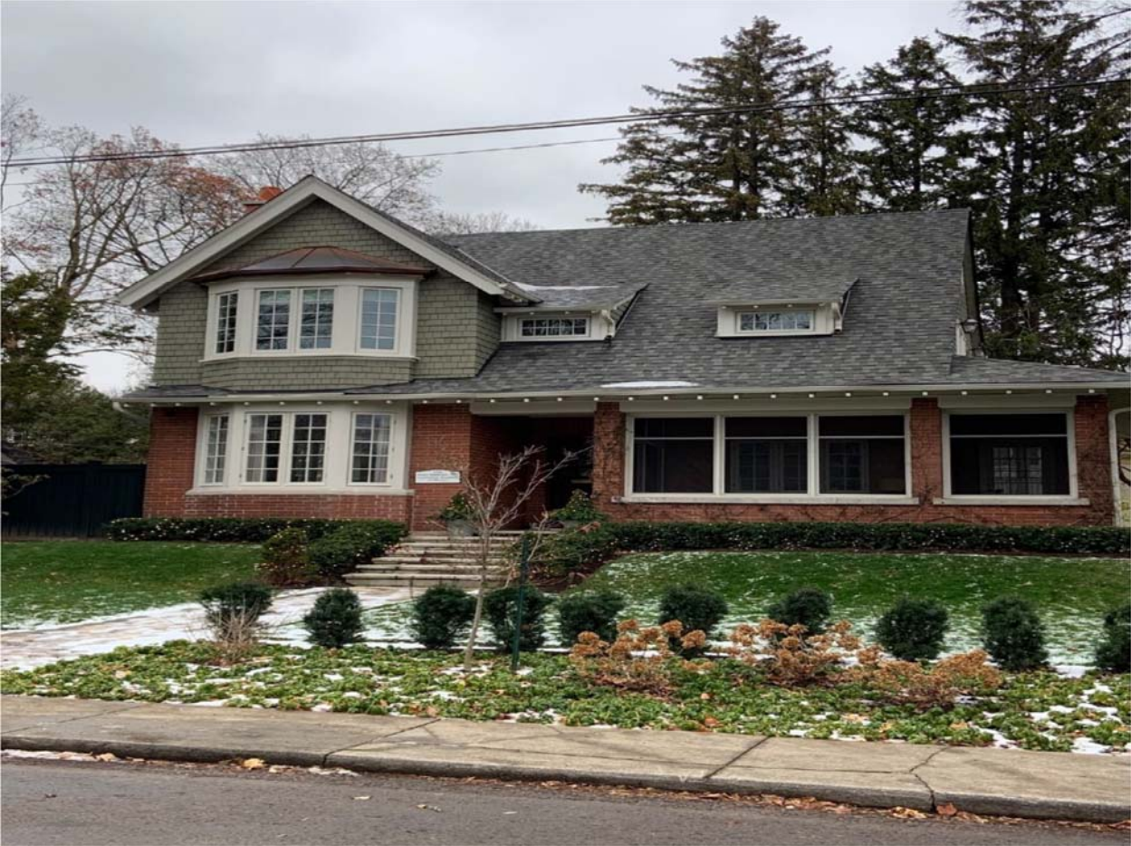
43 Trafalgar Road – Combination Brick and Shake Siding with asphalt roof
