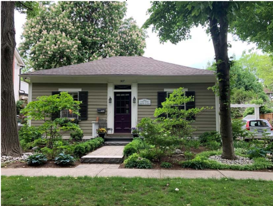
307 William Street – Example of Horizontal Wood Cladding
