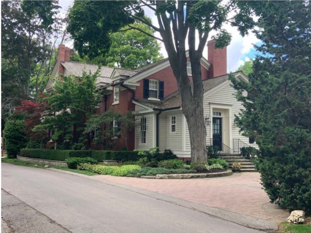
19 Navy Street – addition to rear and visible from side street; height of addition steps down; consistency in roof form and style of windows/doors and trim; complementary use of materials including brick and horizontal wood cladding
