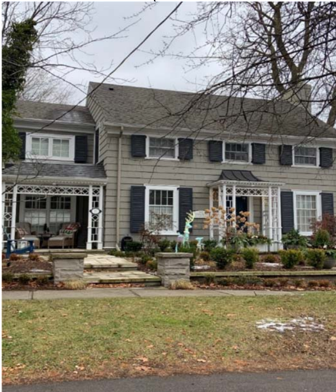
27 Reynolds Street – Asphalt Gable Roof with Shake Cladding
