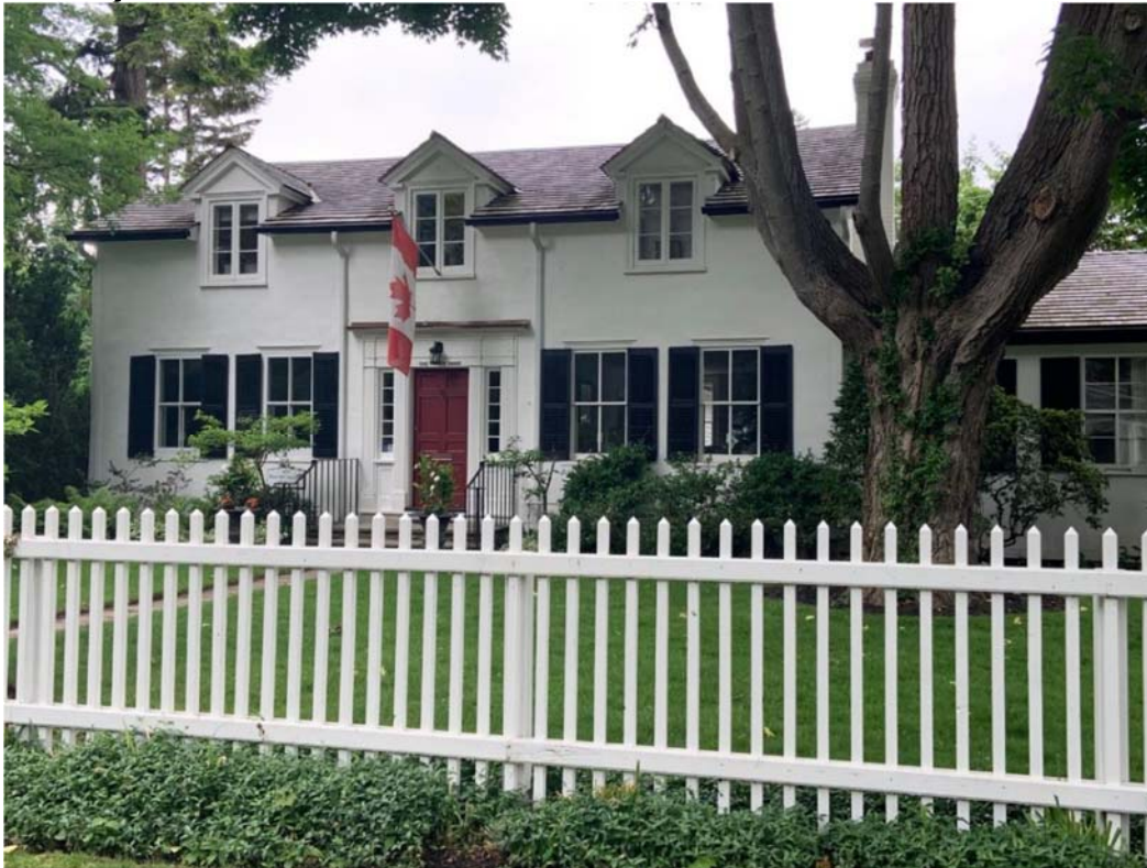
143 Front Street – Cedar Shake Gable Roof with Dormers & Stucco Cladding
