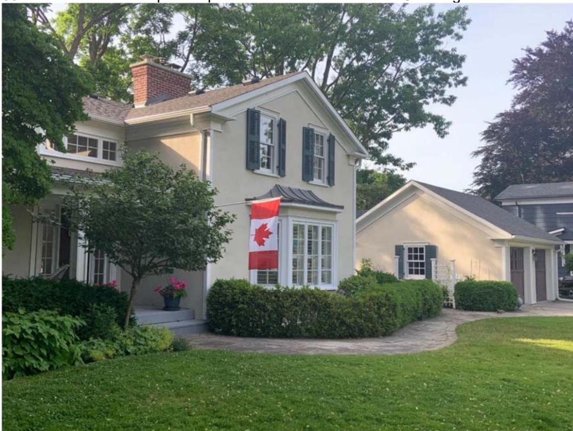
65 Navy Street – Asphalt Gable Roof on House and Garage with Stucco Cladding
