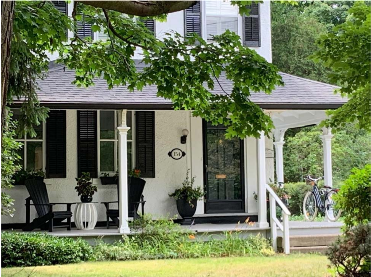
154 King Street – Open Wrap Around Porch
