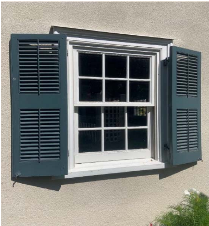
65 Navy Street – Wood Windows with Thermal Pane and Operating Louvered Shutters
