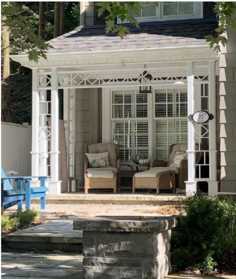
27 Reynolds – Covered Porch
