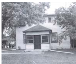
I. 2477 Bronte Road, c. 1870, demolition date unknown.
