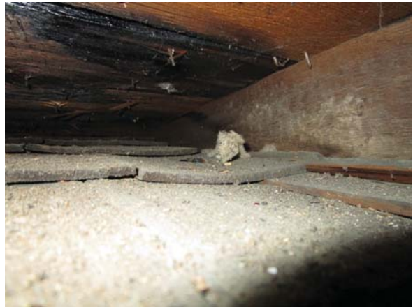
Early roof shingles visible enclosed within the rear structure (ERA, 2018).
