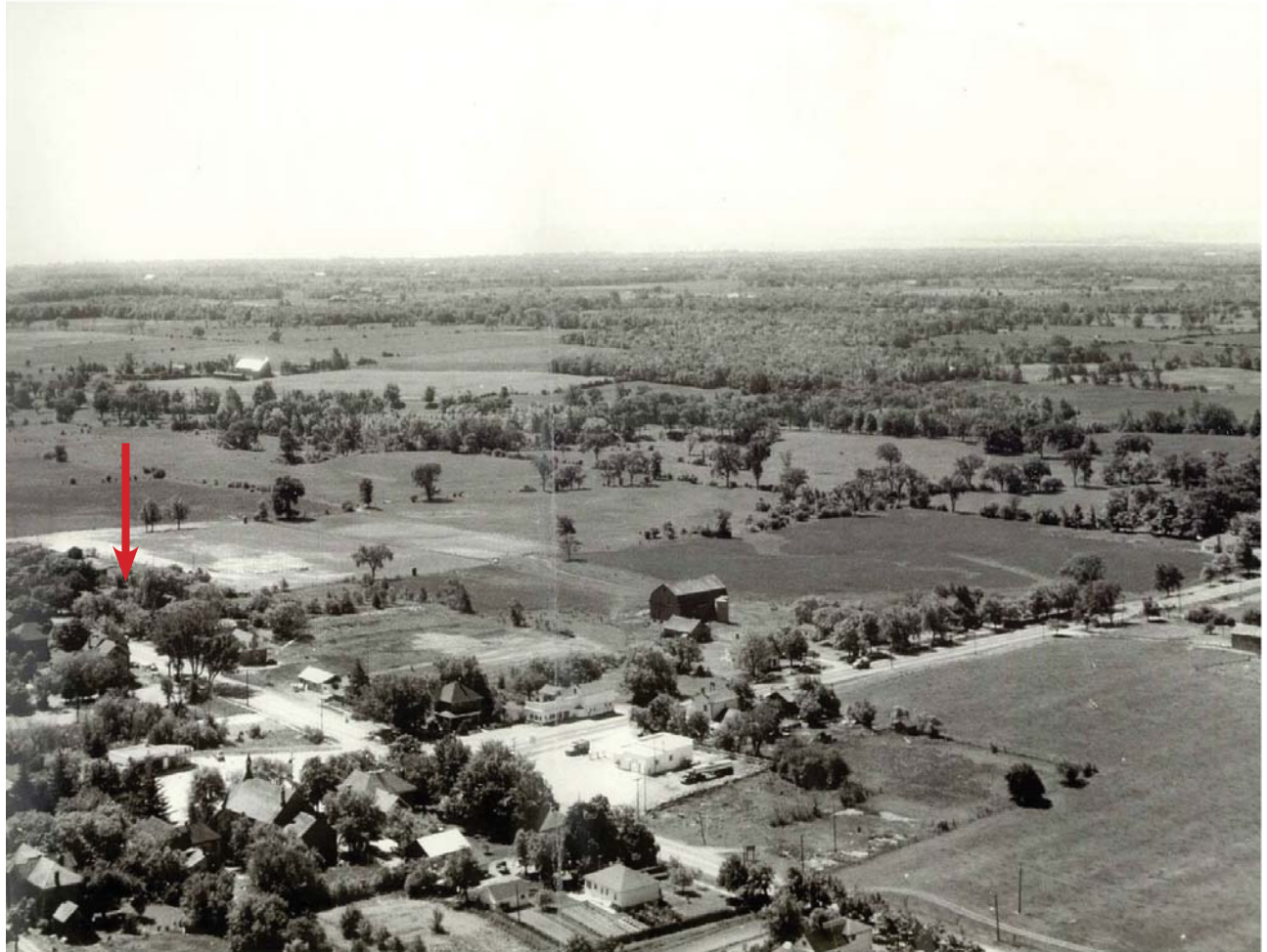
Aerial view looking south-west c. 1950, arrow identifying approximate location of Site (Town of Oakville, annotated by ERA).
