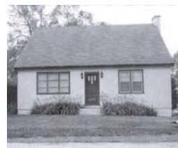
D. 3004 Dundas St., c. 1913, appears to have been relocated (TTHS).
