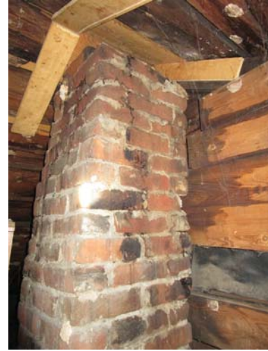
Earlier chimney visible in between the ceiling and roof (ERA, 2018).
