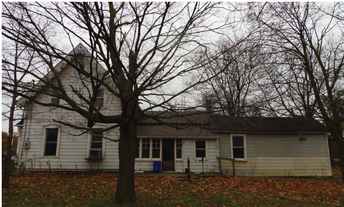
North elevation showing various extensions to the rear of the building (ERA, 2017).
