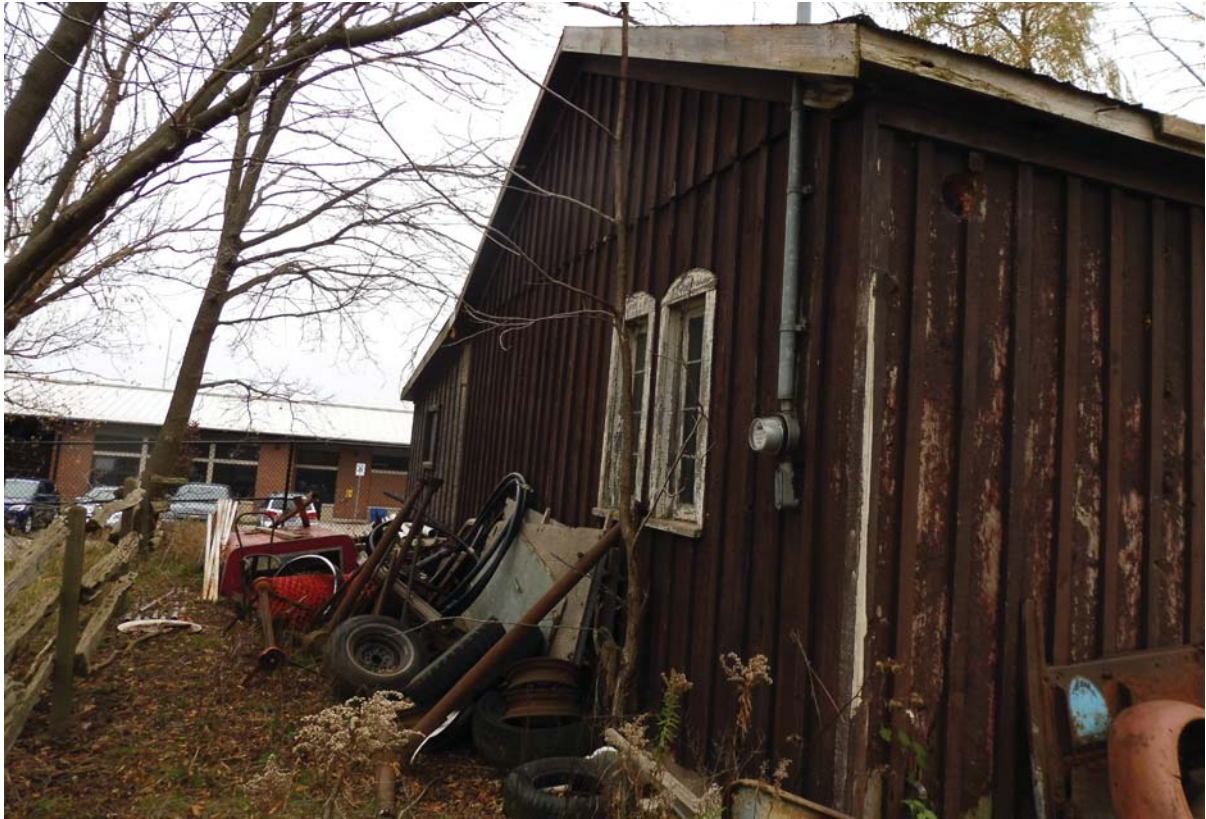
South elevation (ERA, 2017).
