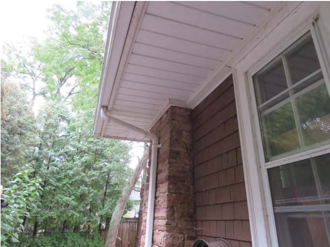
Roof overhang – vinyl siding installed over original wood soffit
