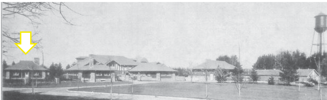
LISONALLY FARM – the Farm Manager’s House was part of a group of farm buildings designed by Page & Warrington
