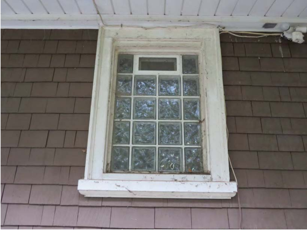
Original window frame with later glass block
