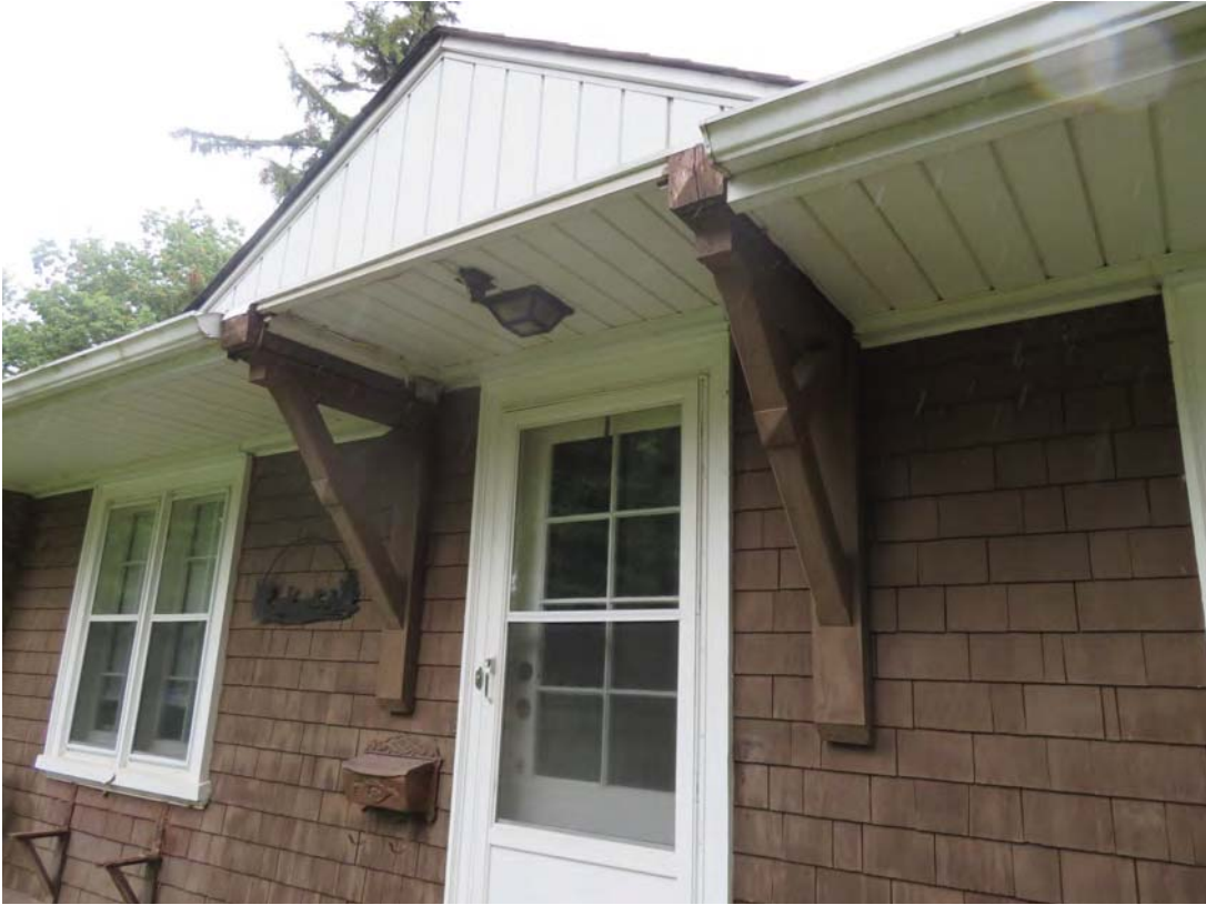
Main entrance - vinyl siding covers original wood soffit and pediment
