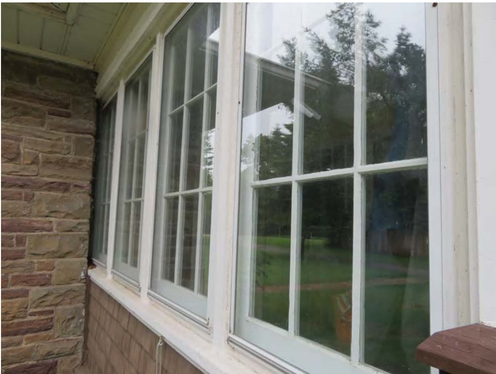
Sunroom wall extends behind the masonry corner pier
