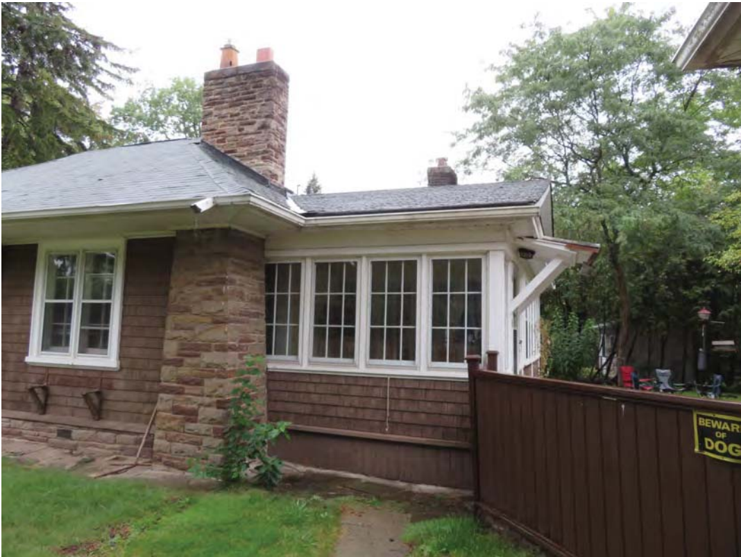
Main elevation – stone chimney
