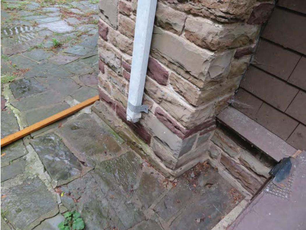
Flagstone paving – quarry cut Credit Valley sandstone
