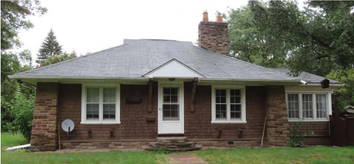
MAIN ELEVATION – oriented towards the driveway
