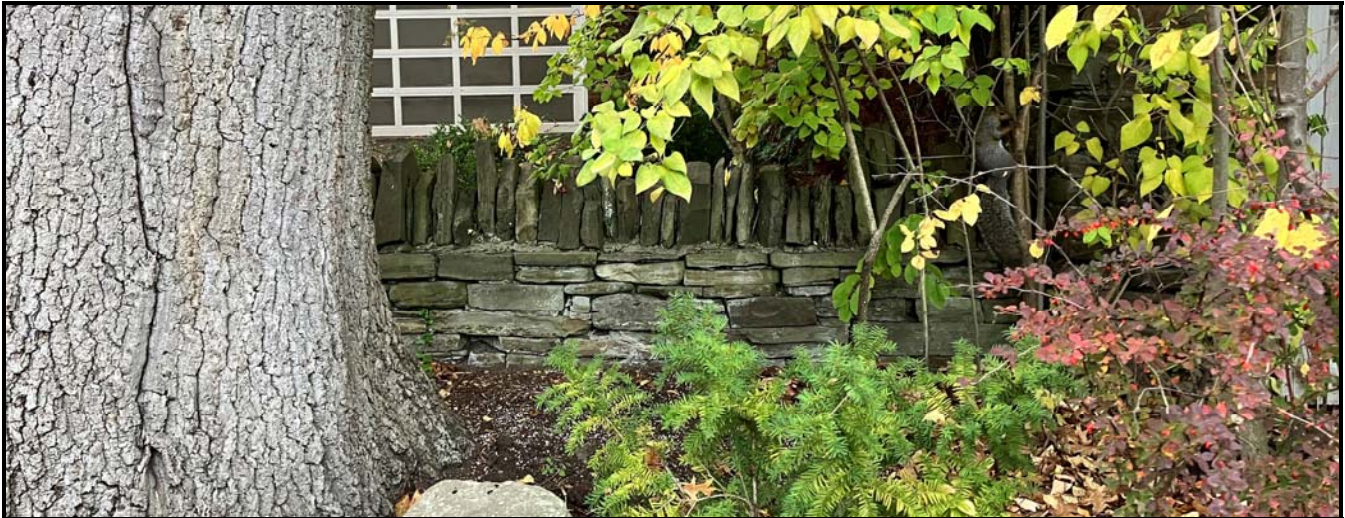
Close up of the dry-laid stone in front of 323 Douglas Avenue, 2024. Source: Town of Oakville Planning and Development Staff
