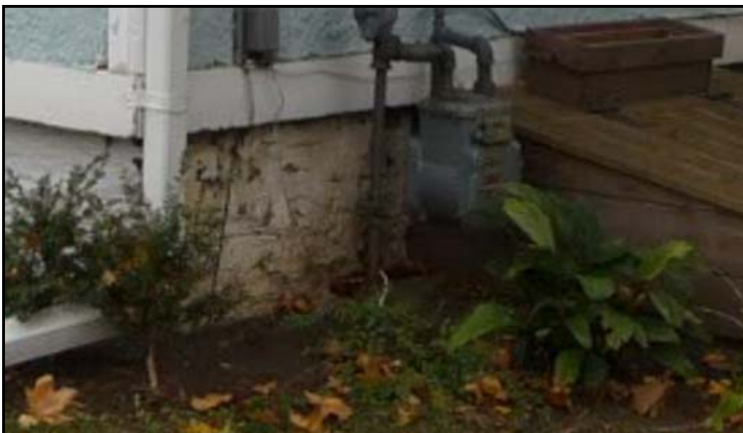
Close-up of the lakestone foundation, partially parged over. Source: Planning Services staff photo, 2008.
