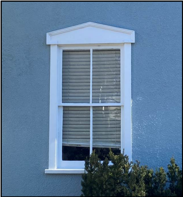
Left: Close up of one of the windows. This one does not have its storm window, but we can see the wooden sash, the pediment, and wooden frame. Source: Planning Services staff photo, 2024.
