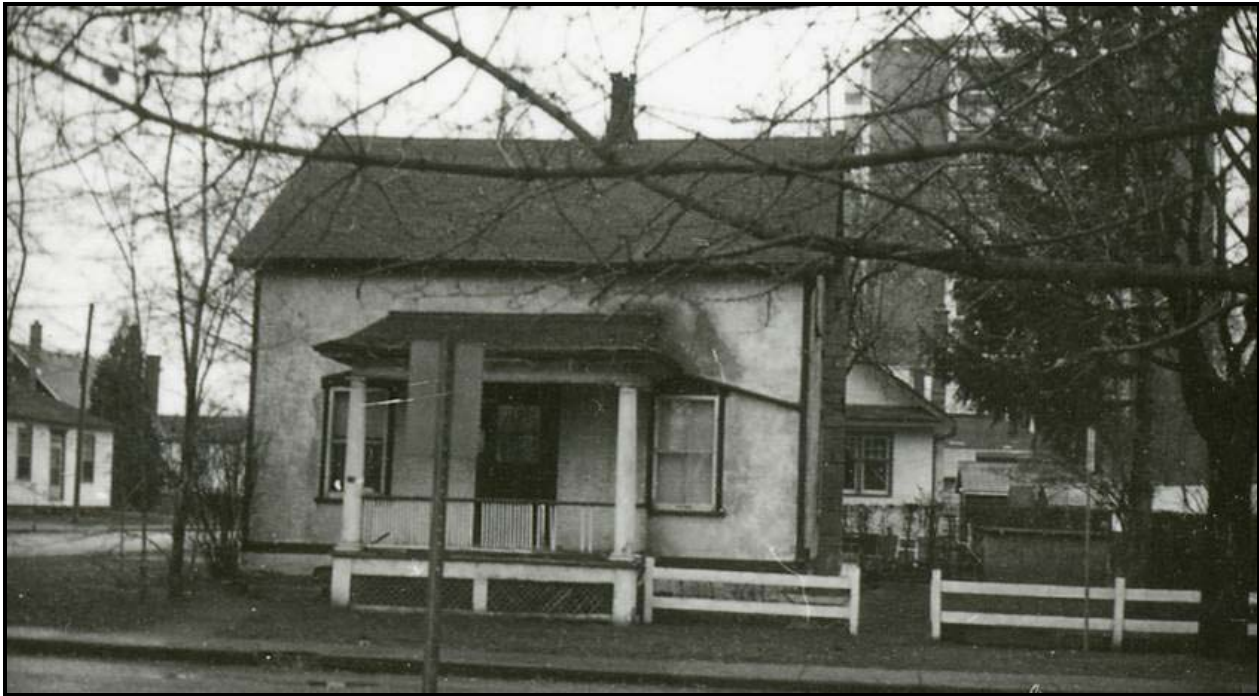
1971 photo showing the historic Neoclassical porch on the front façade. A central chimney was also present on the roof and was likely removed later. Note the wooden trim on each corner of the house and along the foundation that is still present. Source: Canadian Inventory of Historic Buildings, Parks Canada.
