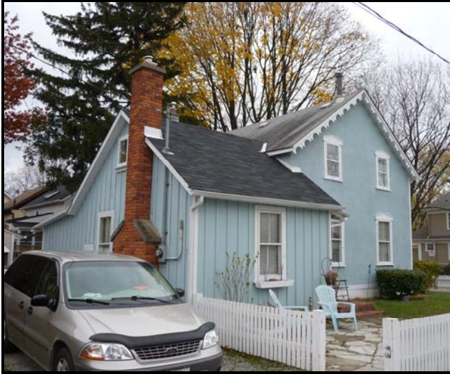
Left: 2008 image of the rear wing. Source: Planning Services staff photo.
