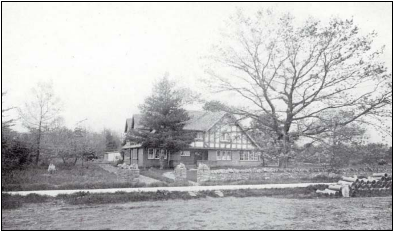
1913 image of the house, showing original elements that still stand, including the lakestone wall and columns. Source: 1913 Brantwood promotional booklet, Cumberland Land Company Ltd. and W.S. Davis
