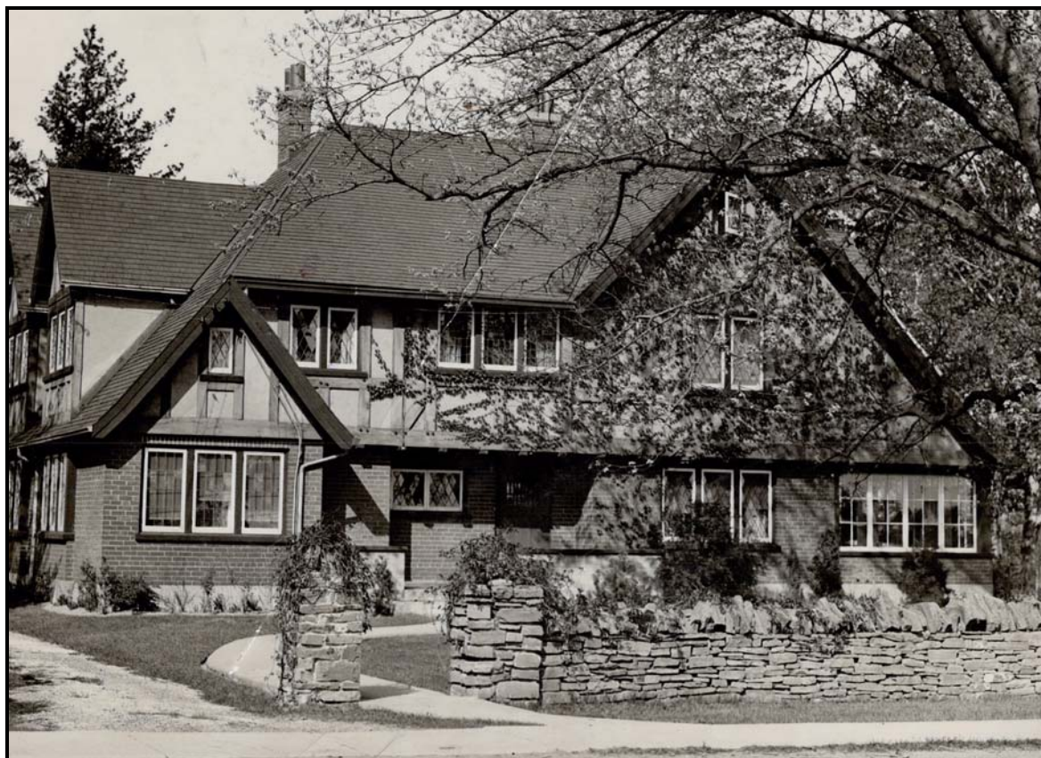
Photo of the house in 1929, published in the Toronto Star . Source: Toronto Public Library – Toronto Star Photograph Archive
