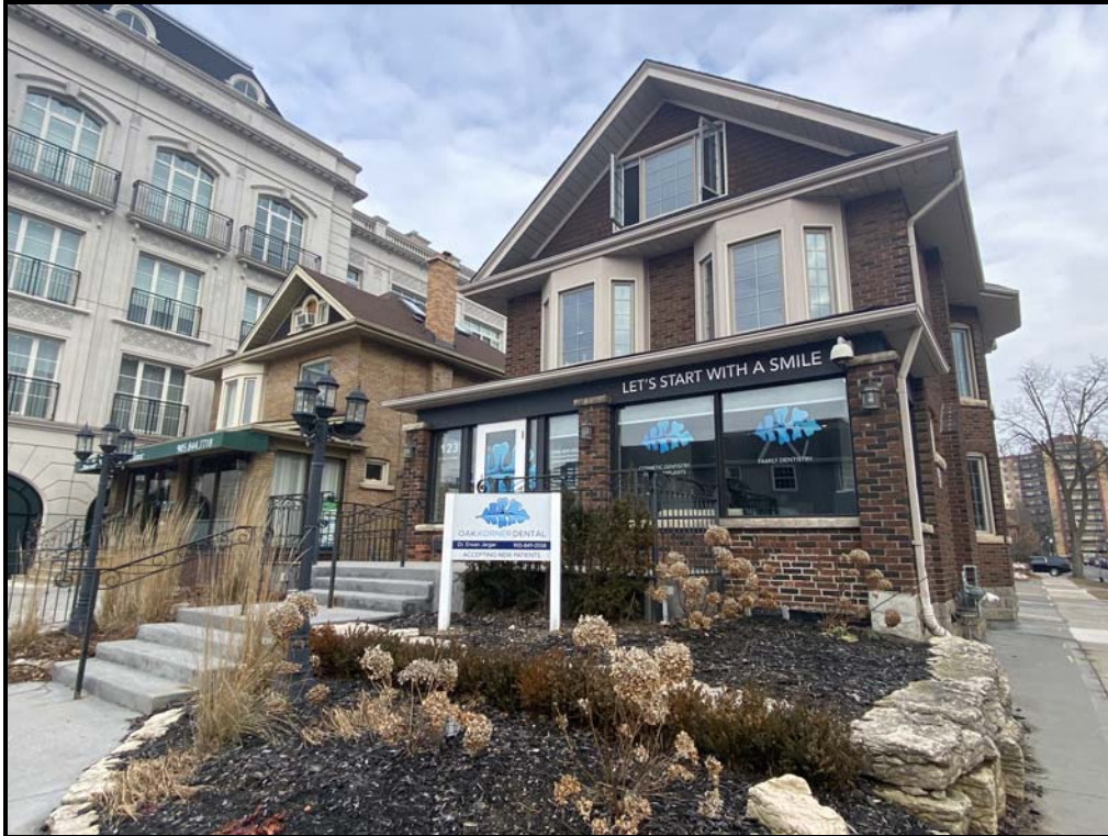
West (front) elevation of the building, 2024. Source: Town of Oakville Planning Services Staff
