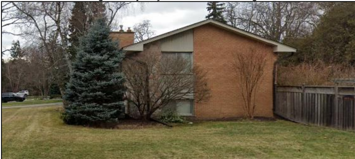
Existing Flankage Yard – 1291 Cambridge Drive
