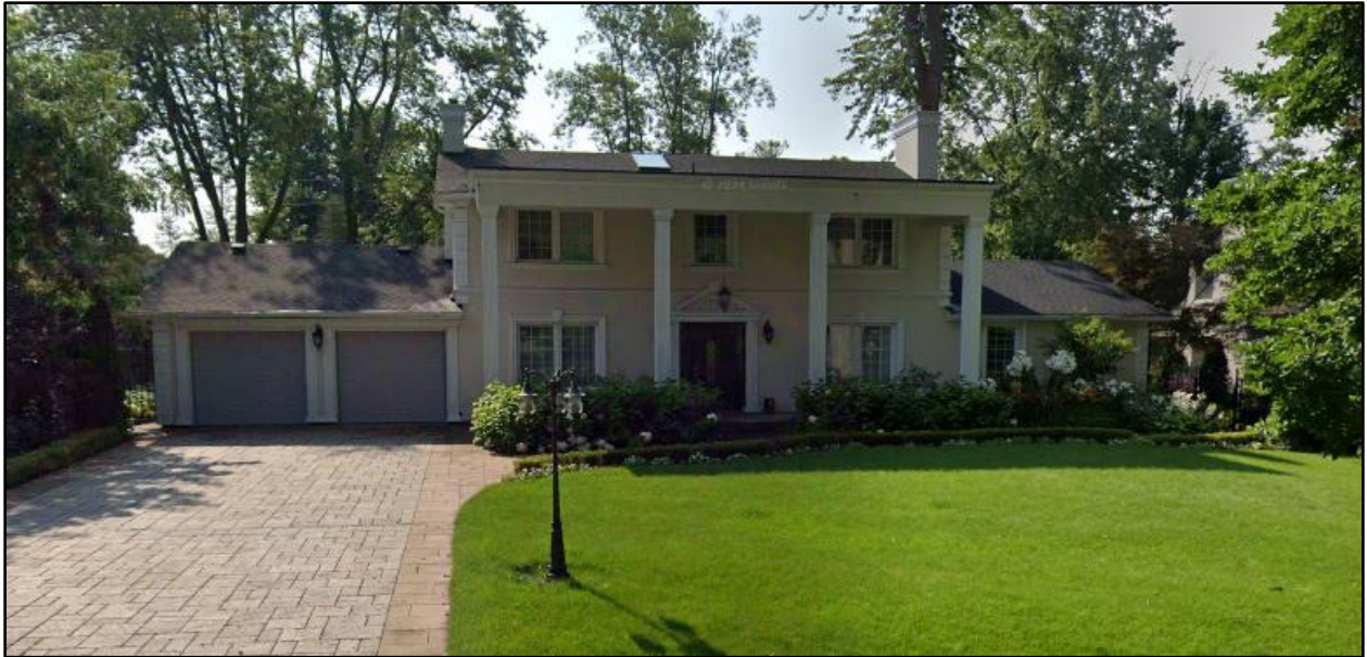
Primary Façade – 1316 Cambridge Drive (east of Cairncroft Road)
