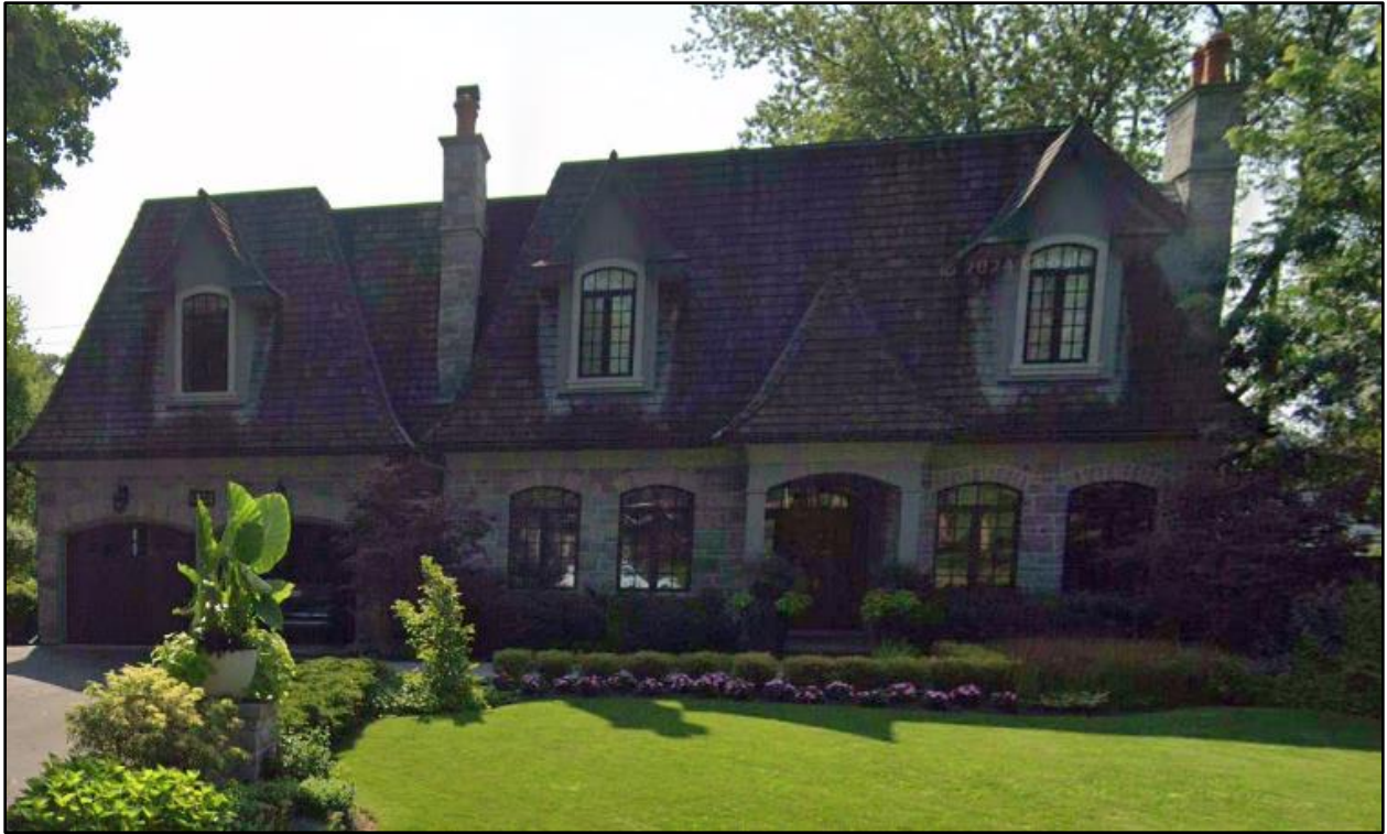
Primary Façade - 1324 Cambridge Drive (east of Cairncroft Road)
