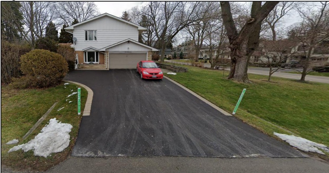
Flankage Condition – 1305 Cambridge Drive (across from subject lands)
