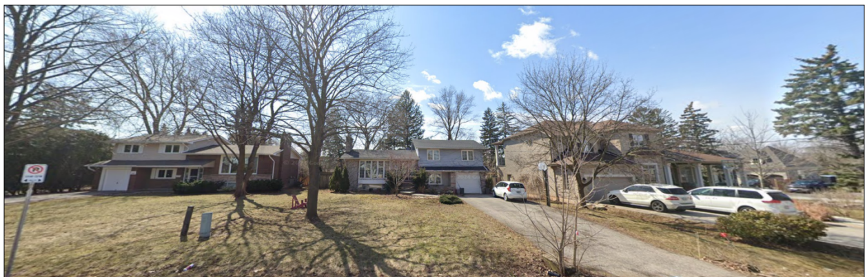
Street View of 324 Wendy Lane
