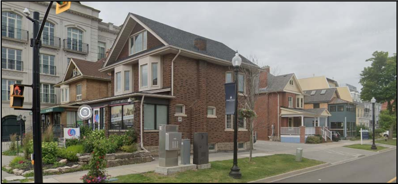
2024 view looking northeast from Trafalgar Road and Church Street, with the subject property in the foreground. Source: Google
