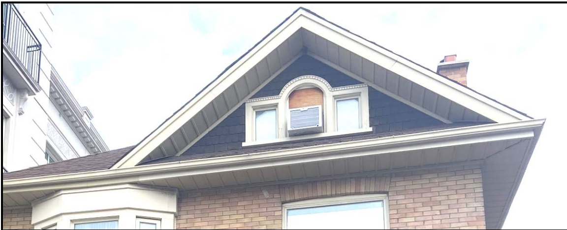
Fish scale cladding on the gable. Source: Town of Oakville Planning and Development Staff
