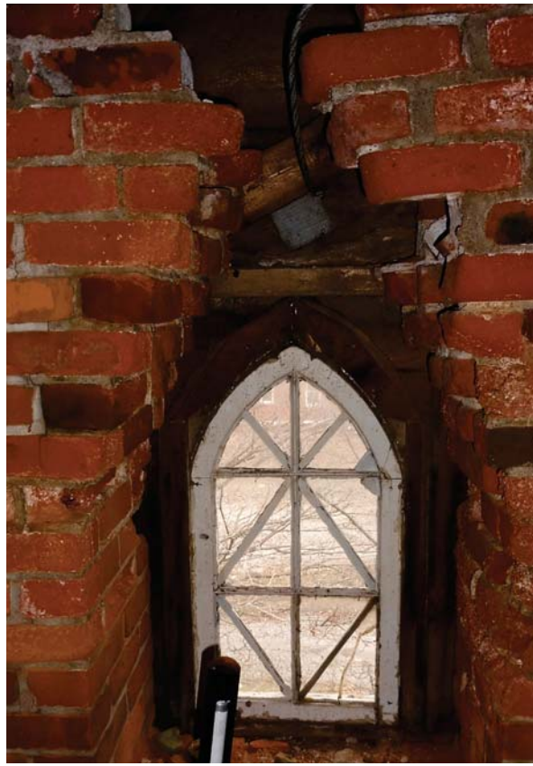
Showing original lancet window in attic in good repair, and brickwork in poor condition (ERA, 2017).
