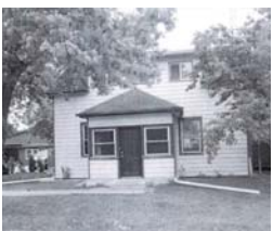
I. 2477 Bronte Road, c. 1870, demolition date unknown.
