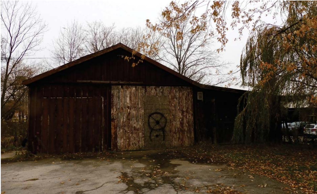
North elevation (ERA, 2017).
