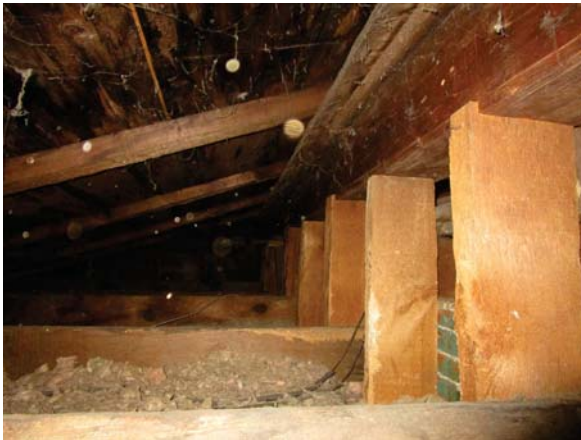
Early roof structure enclosed within a new roof structure(ERA, 2018).
