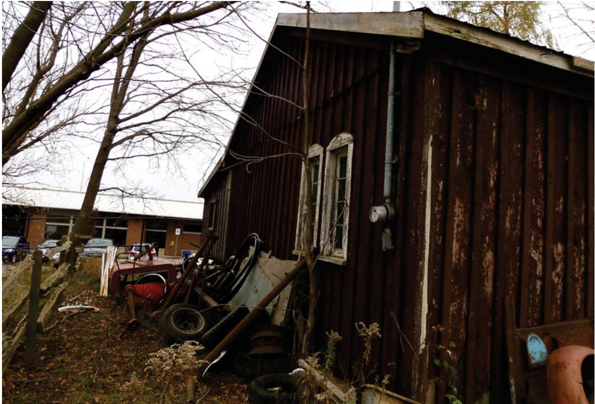
South elevation (ERA, 2017).
