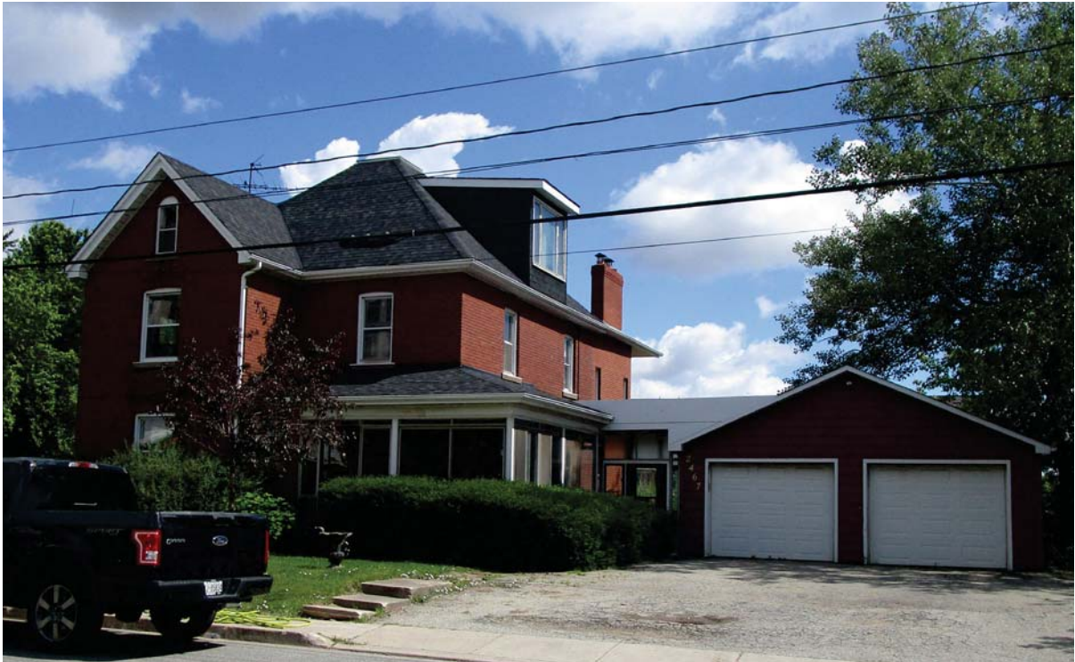
2467 Old Bronte Road (ERA, 2017).
