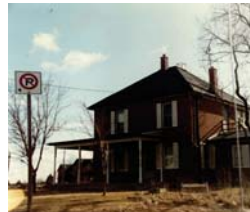
C. 2496 Bronte Rd., c. 1945, demolition date unknown.
