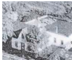
F. Dundas St., c. 1860-70s, possible second Smith farmhouse, demolition date unknown.
