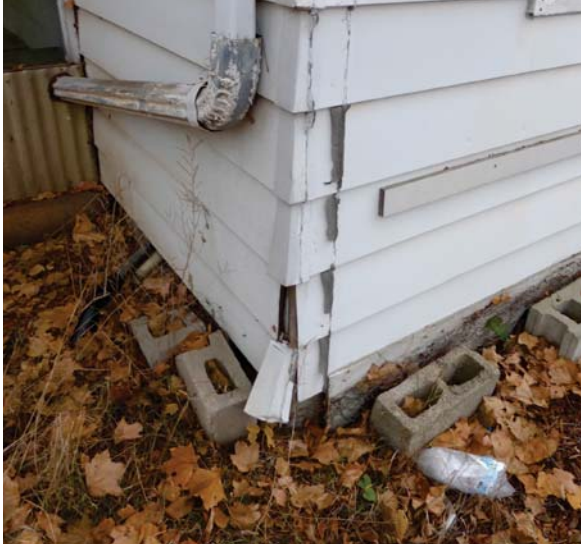
Showing wood rot to cladding substrate and sections of vinyl siding in poor condition (ERA, 2017).
