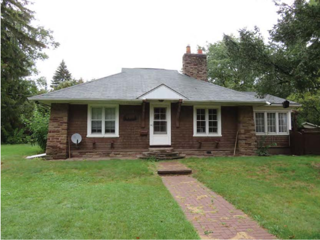
Walkway to main entrance
