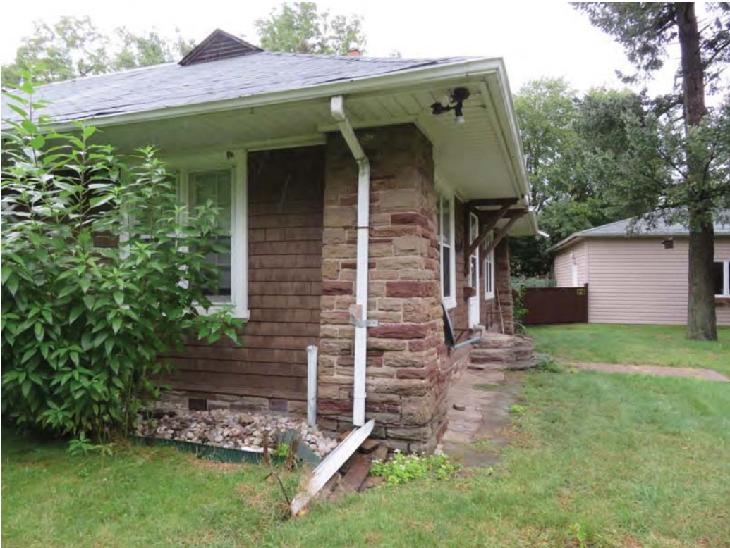
Masonry piers at the corners are flared – wide roof overhang – eyebrow dormers in the low hipped roof
