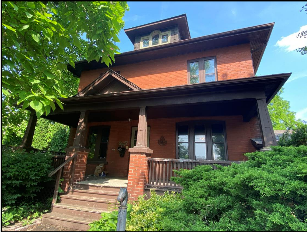
South elevation (front façade).
