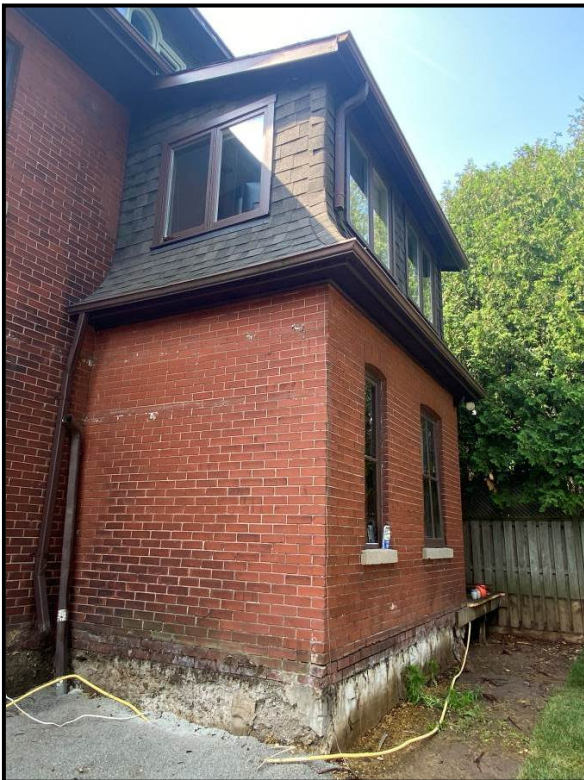
East and north elevation of the rear wing.
