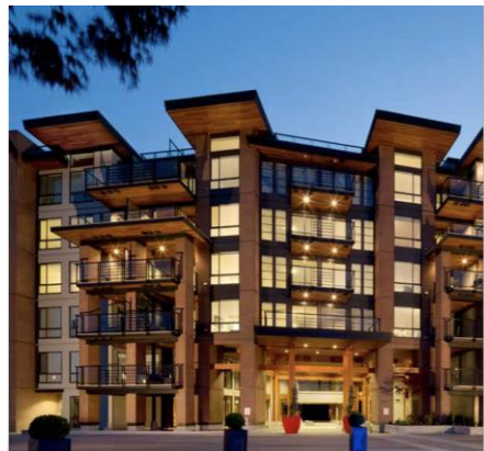
The Shore, North Vancouver, BC. Wood Frame 6 storey. Adera Development Corporation As shown in Mid Rise Best Practice Guide, BC Housing
