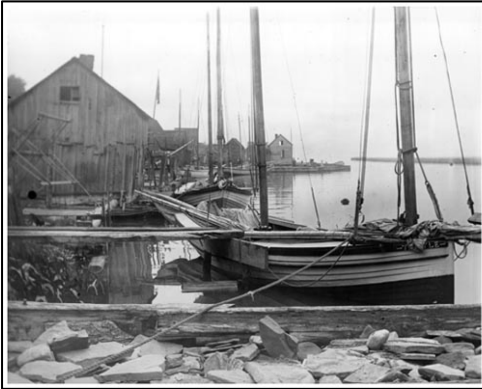
Bronte Harbour, 1910. Source: Town of Oakville Heritage Planning files.
