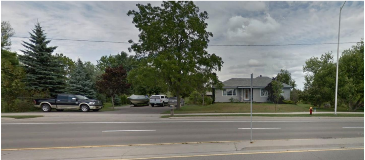
Figure 5. 1477 Burloak Drive – Existing conditions
