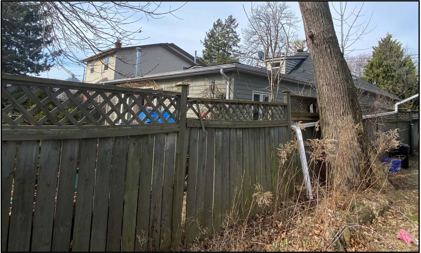
View of the rear of the house, taken from the rear yard of 2374 Sovereign Street, 2024. Source: Town of Oakville, Planning Services staff photo
