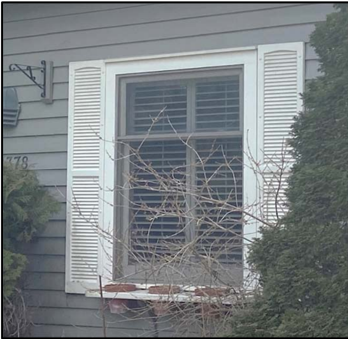
Close-up of one of the historic 1/1 wood sash windows, 2024. Source: Town of Oakville, Planning Services staff photo
