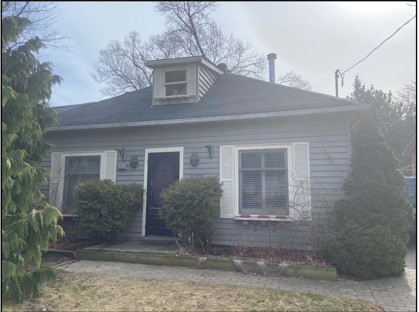
Front elevation of the house, 2024. Source: Town of Oakville, Planning Services staff photo
