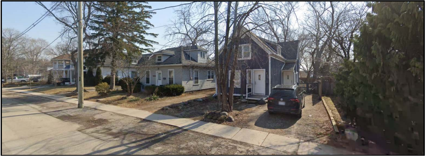
Looking southeast towards 2374 Sovereign Street. March 2022. Source: Google Street View
