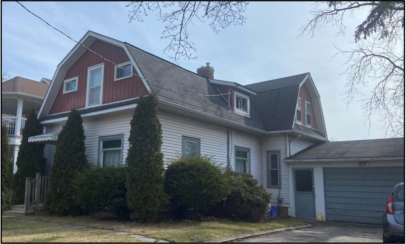
Front and west elevations of the house, 2024. Source: Town of Oakville, Planning Services staff photo
