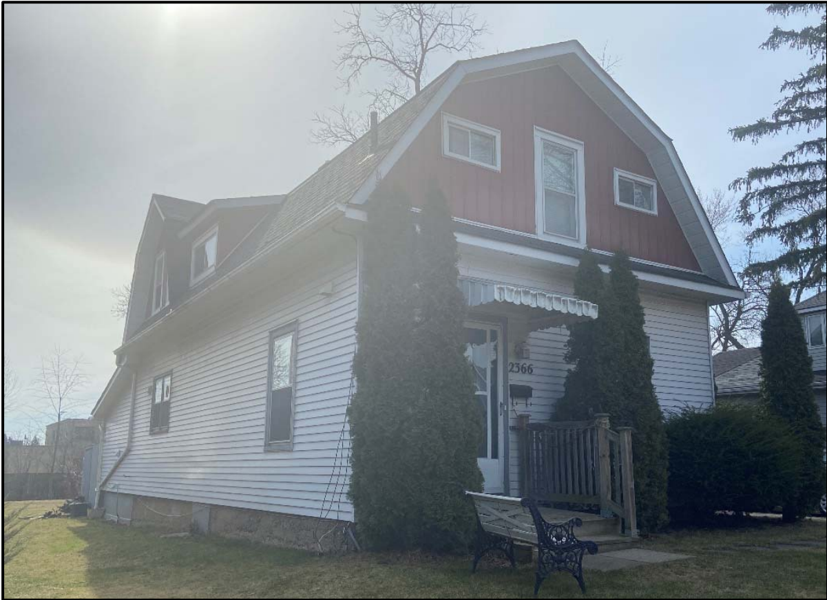
Front and east elevations of the house, 2024. Source: Town of Oakville, Planning Services staff photo
