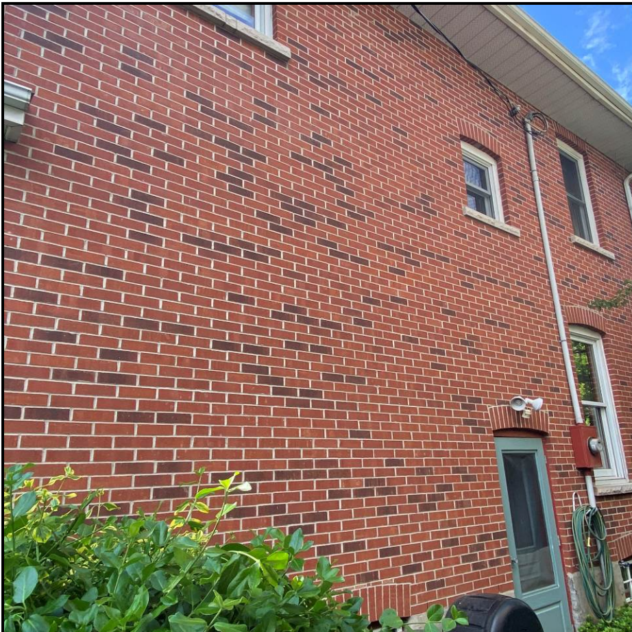
Close-up of the running bond brick pattern, 2024. Source: Town of Oakville Planning Staff
