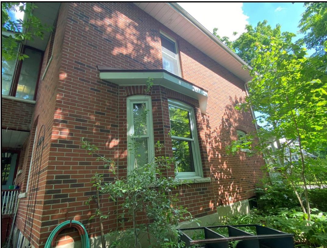
Bay window on south elevation with two other windows, 2024. Source: Town of Oakville Planning Staff
