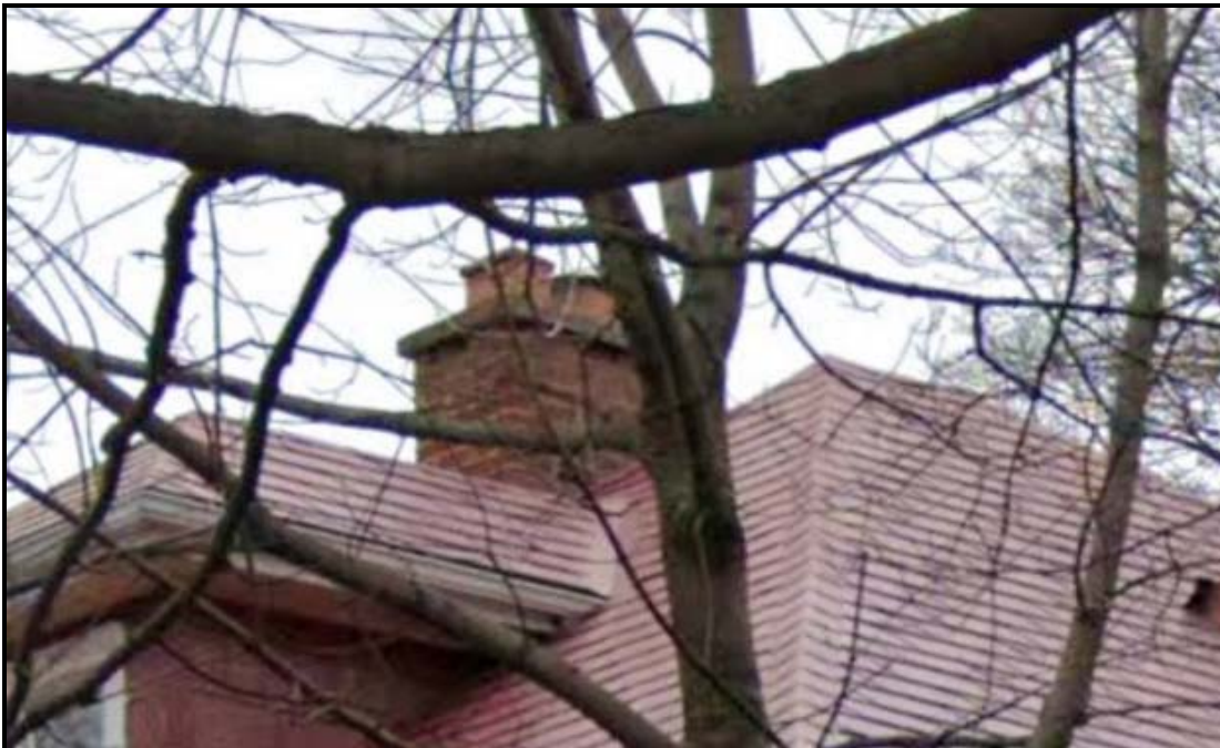
Close-up of the brick chimney, 2021. Source: Google
