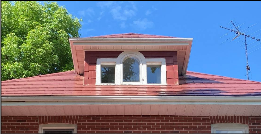
Palladian window in the front dormer, 2024. Source: Town of Oakville Planning Staff
