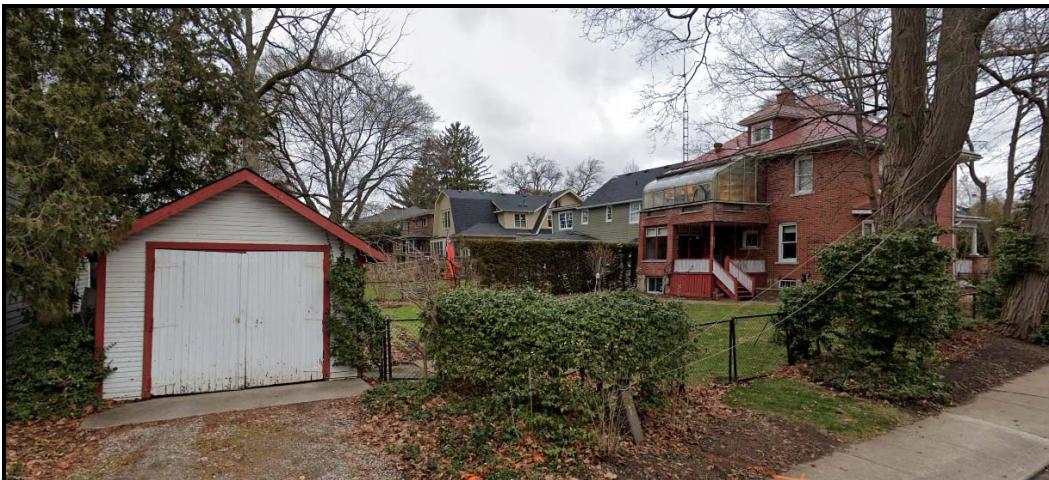
Original frame garage on the property, 2021. Source: Google
