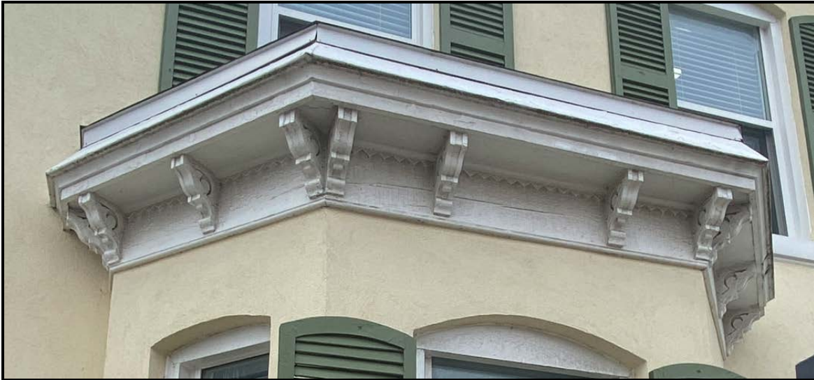
Close-up of the projecting bay window wooden detailing, 2024. Source: Town of Oakville Planning Staff
