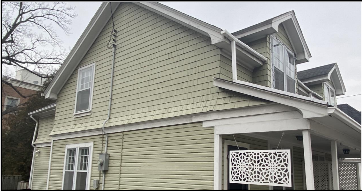
Bell-cast overhang of adjacent house at 131-135 Chisholm Street, 2024. Source: Town of Oakville Planning Services Staff
