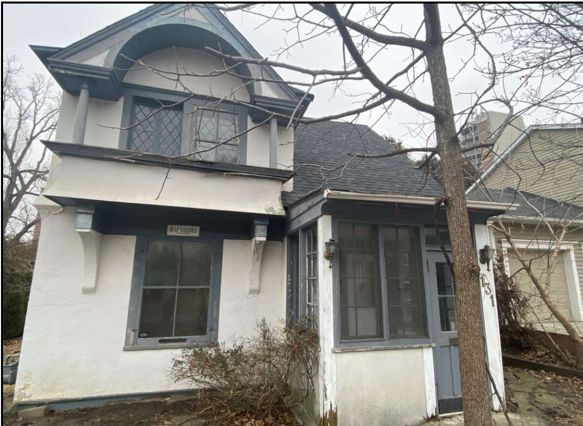
West elevation (front), from Chisholm Street, 2024. Source: Town of Oakville Planning Services Staff
