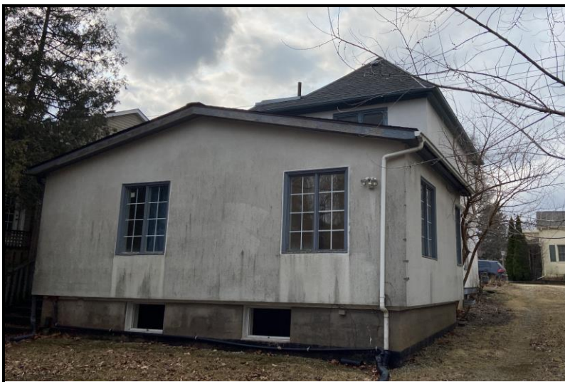
East elevation, showing the rear of the house and a later addition, 2024. Source: Town of Oakville Planning Services Staff
