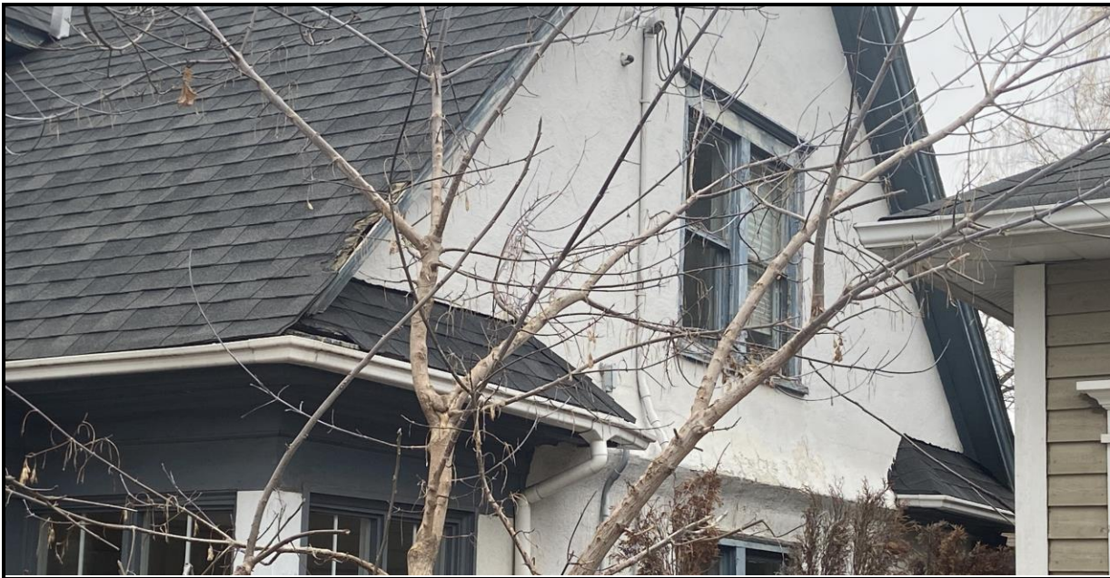
Side gable roof on the south elevation with roof-style returns, 2024. Source: Town of Oakville Planning Services Staff
