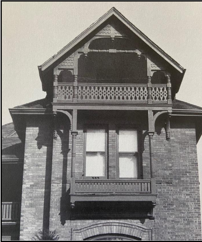
An example of a similar, yet more elaborate, second storey balcony with gable roof on a Queen Anne style house. Source: Ontario Architecture by John Blumenson.
