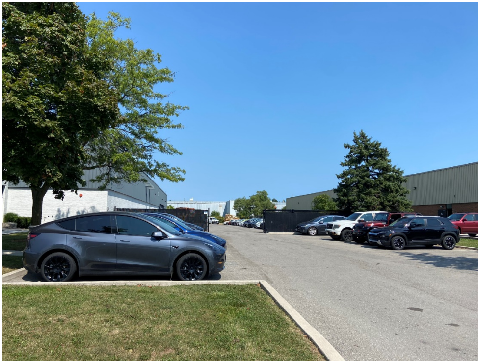
View of the Motor Vehicle Storage Compound from the edge of the subject property, taken on September 5, 2024
