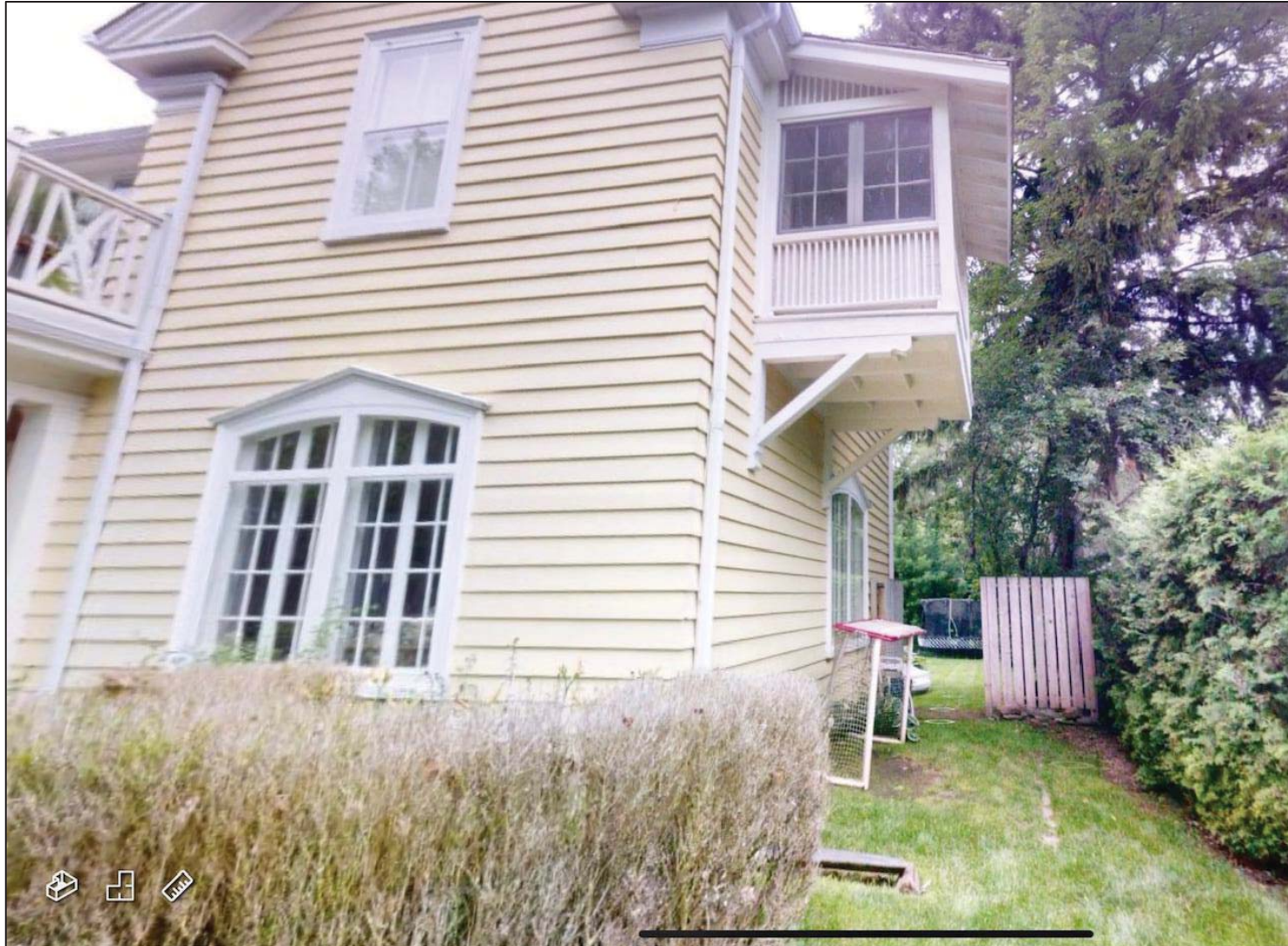
31 FIRST STREET - PORCH ADDITION PHOTO OF EXISTING HOUSE
