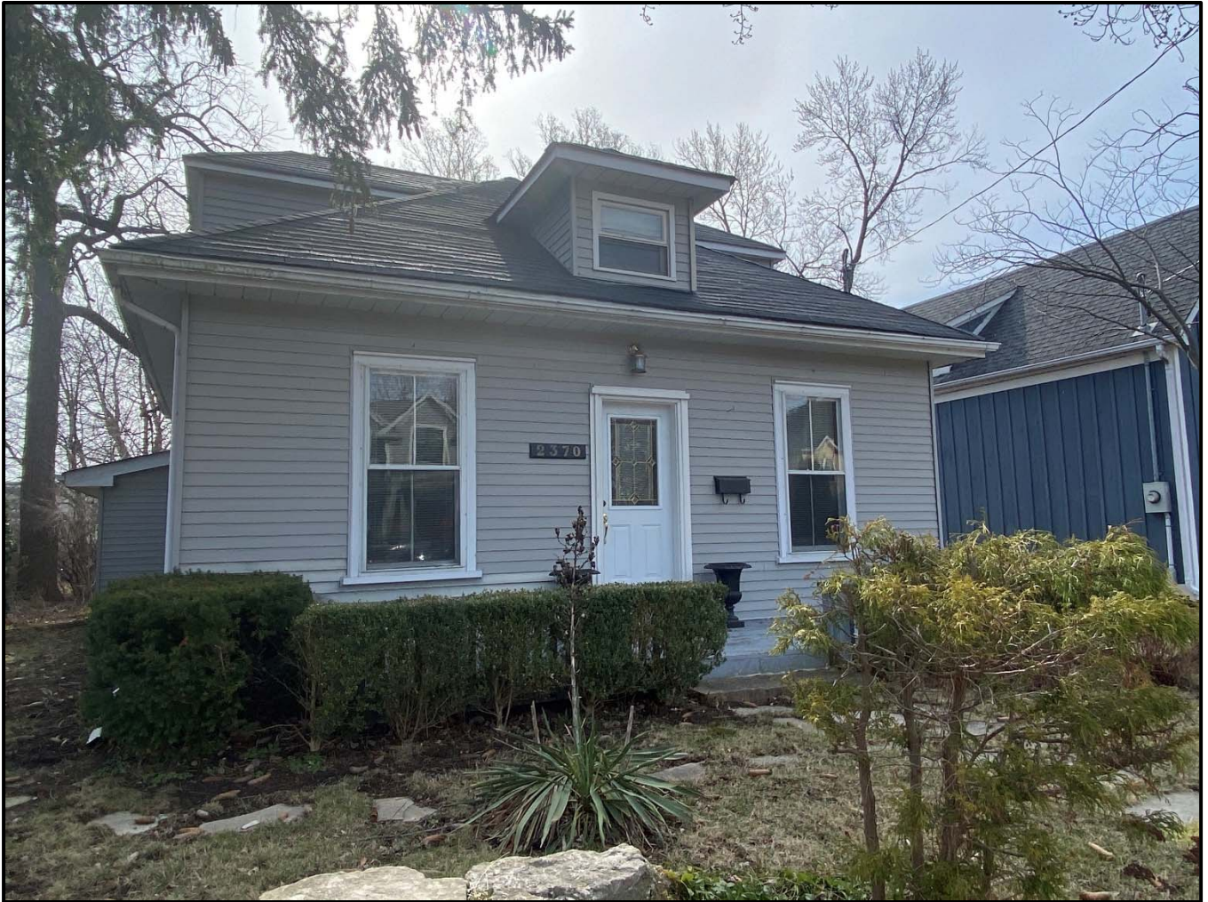
2370 Sovereign Street, 2024. Source: Town of Oakville, Planning Services staff photo
