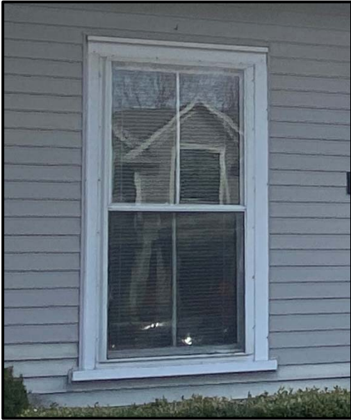
Close-up of one of the historic 2/2 wood sash windows, 2024. Source: Town of Oakville, Planning Services staff photo
