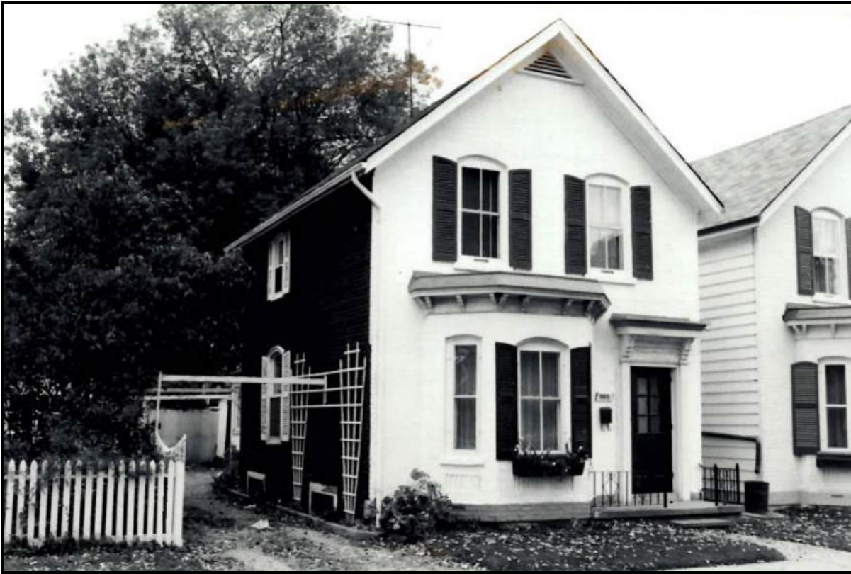
Photo of the subject property, circa 1980s, showing the same windows. Source: Town of Oakville planning files
