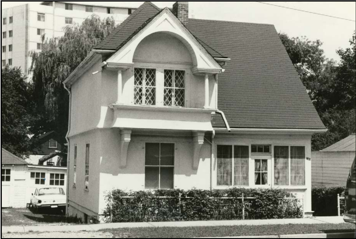
The house circa 1981. Notice the lack of vestibule at the front, and we see the original enclosed porch. The 1980s rear wing is also not present and the property contains a detached garage. Source: Town of Oakville planning files
