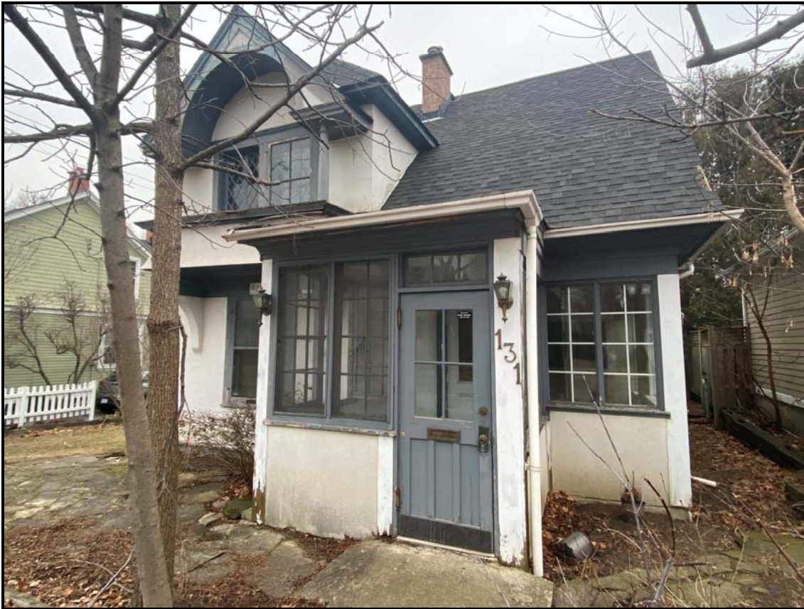
Front vestibule addition with salvaged historic windows, door and transom window. Source: Town of Oakville Planning Services Staff
