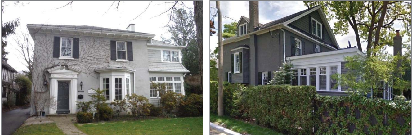
Figure 14: 75 Second St. - an 1850s house with a compatible early 20th century two-storey addition set back to the side of the main elevation (left); 56 Second St. – a 1914 house with a compatible 2002 one-storey addition at the rear of the main structure (viewed from side elevation on Union St.) (right).
