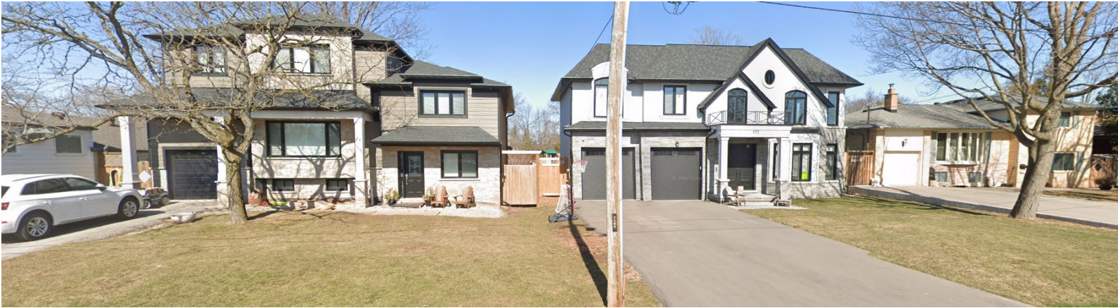
View looking north toward 659, 655 and 651 Trafford Crescent
