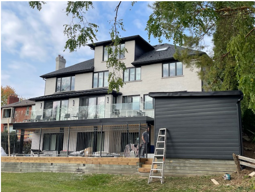
Figure 2 Image of 3232 Shoreline Dr rear yard 2023 after cosmetic work and repairs
