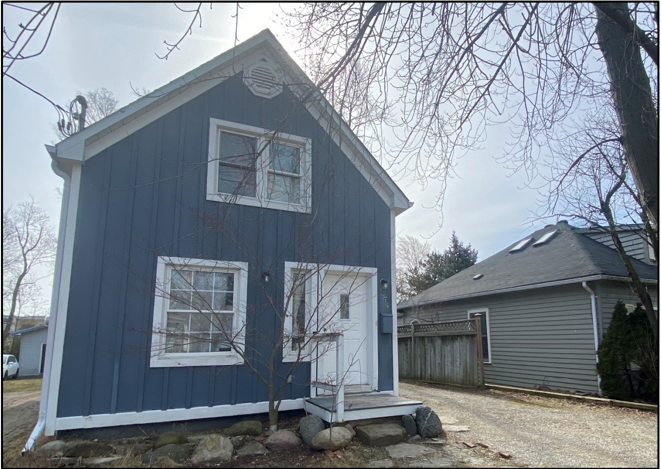
North elevation of the house, 2024. Source: Town of Oakville, Planning Services staff photo
