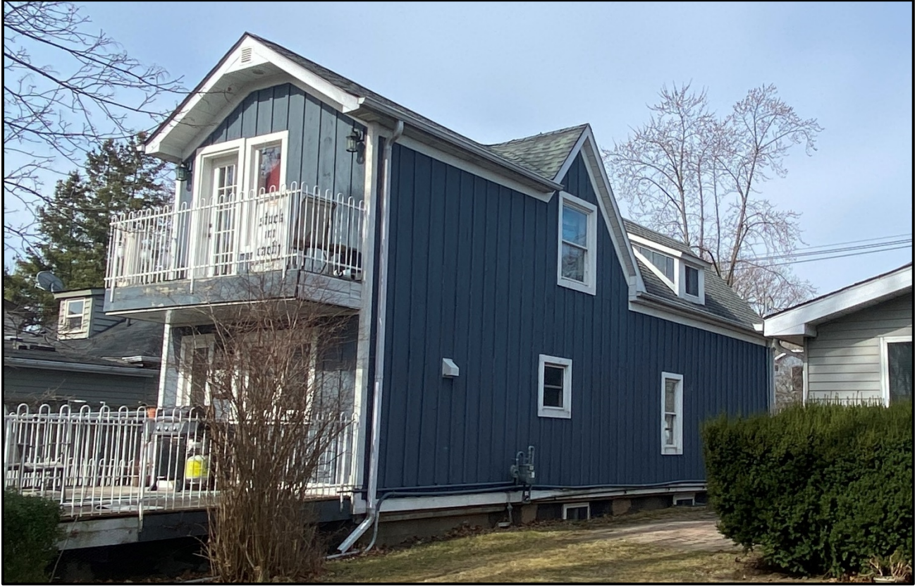
East elevation of the house, 2024. Source: Town of Oakville, Planning Services staff photo
