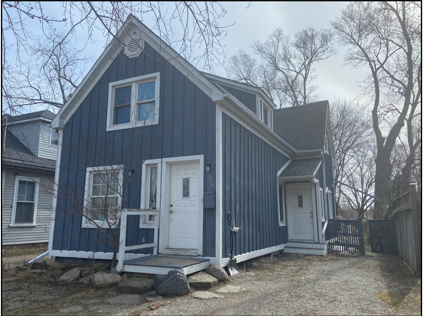
Front elevation of the house, 2024. Source: Town of Oakville, Planning Services staff photo
