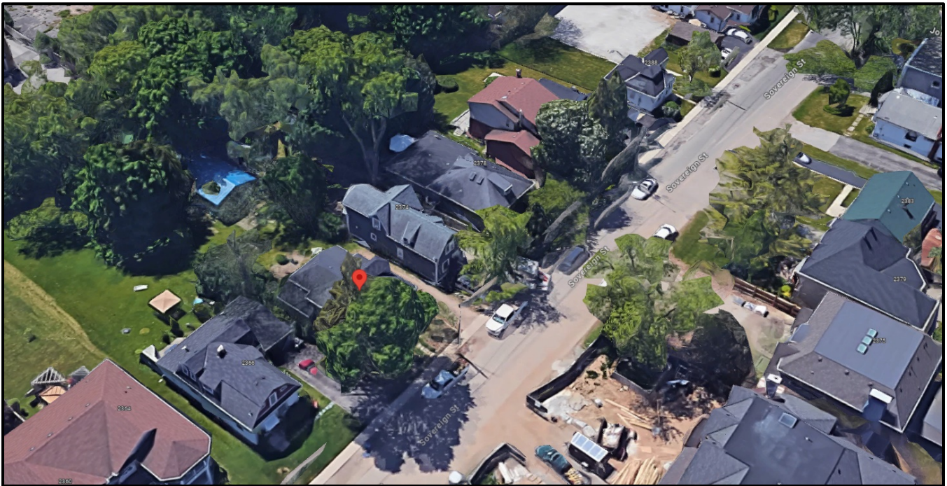
Aerial view of 2370 Sovereign Street. 2021. Source: Town of Oakville, GIS
