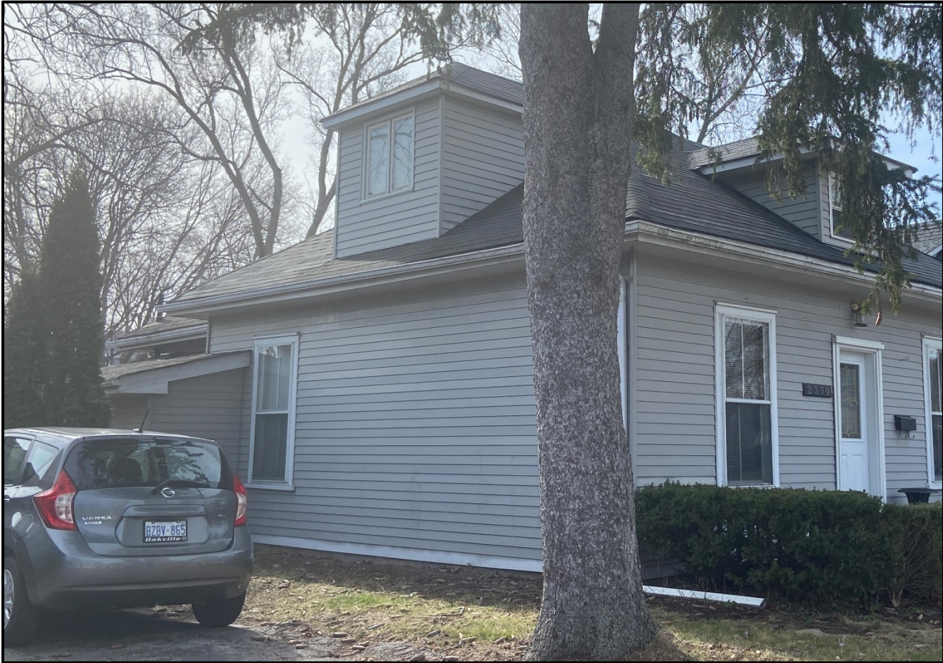
East elevation of the house with contemporary dormer, 2024. Source: Town of Oakville, Planning Services staff photo
