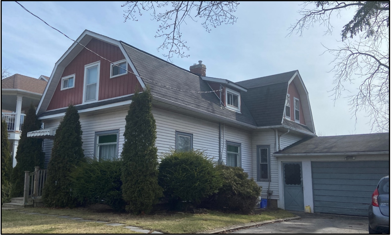
Front and west elevations of the house, 2024. Source: Town of Oakville, Planning Services staff photo
