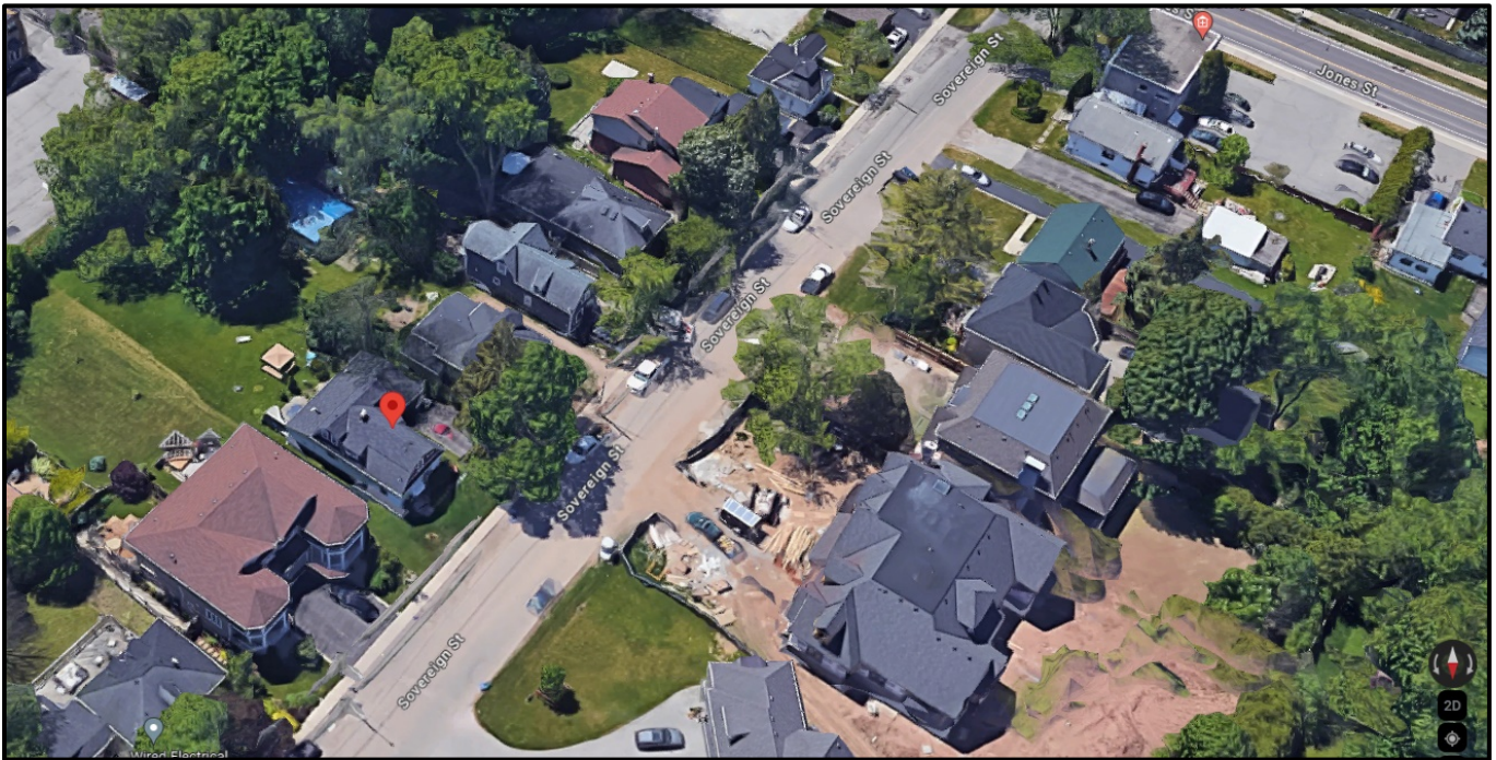
Aerial view of 2366 Sovereign Street. 2021. Source: Town of Oakville, GIS
