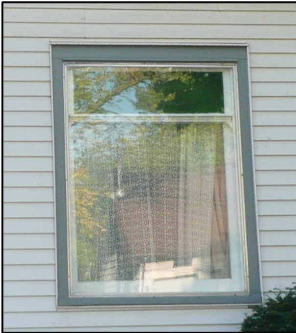
Close-up of one of the historic 1/1 wood sash windows, 2024. Source: Town of Oakville, Planning Services staff photo
