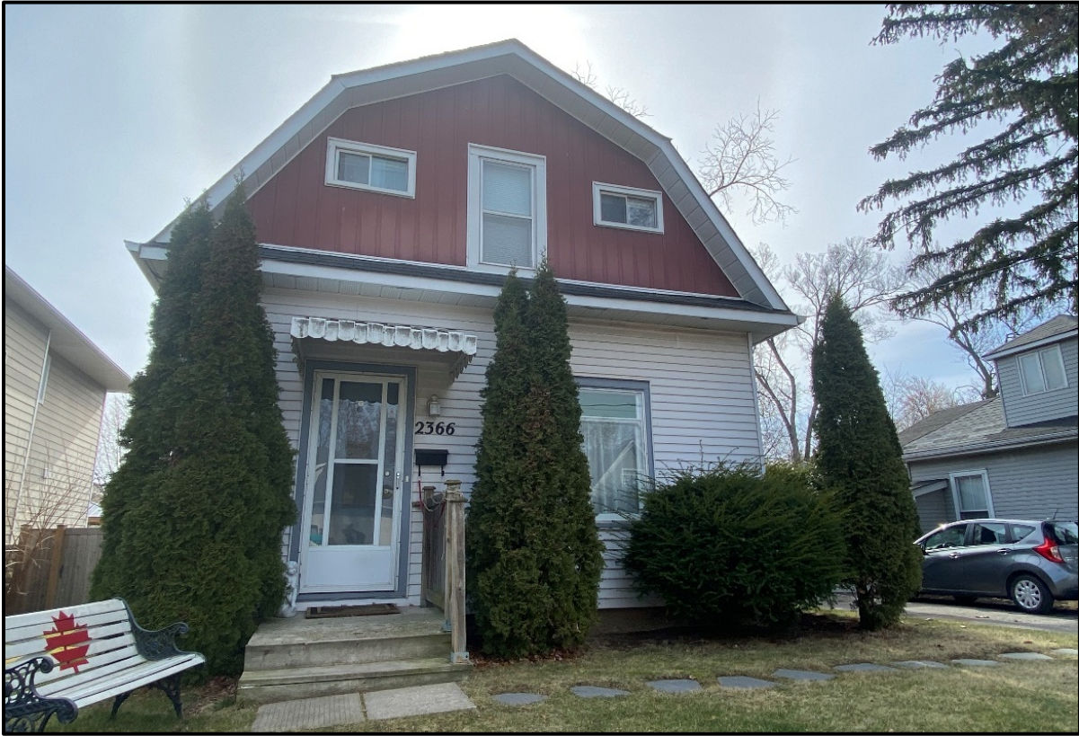
Front elevation of the house, 2024. Source: Town of Oakville, Planning Services staff photo
