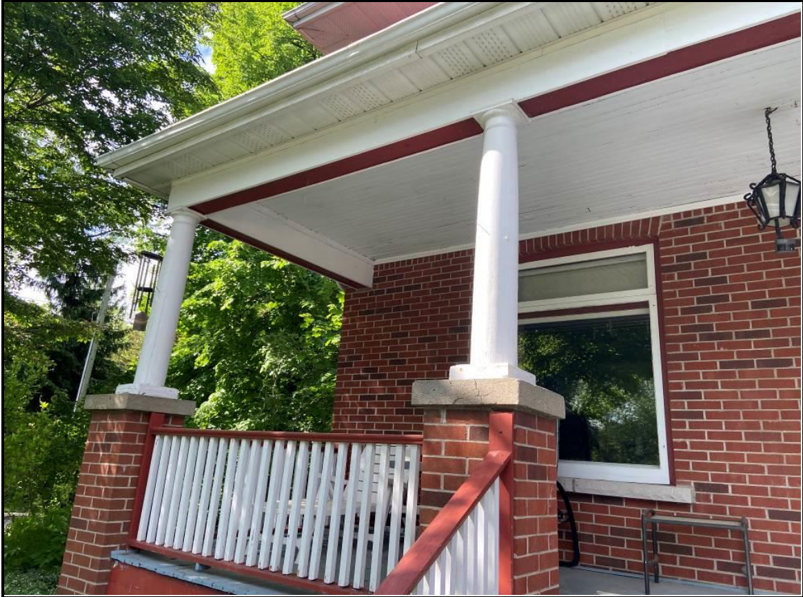
Close-up of two of the columns on brick piers, with the wooden ceiling and wooden architrave, 2024. Source: Town of Oakville Planning Staff
