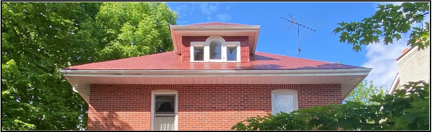
Hipped roof with hipped roof dormer on the east elevation of the house, 2024. Source: Town of Oakville Planning Staff
