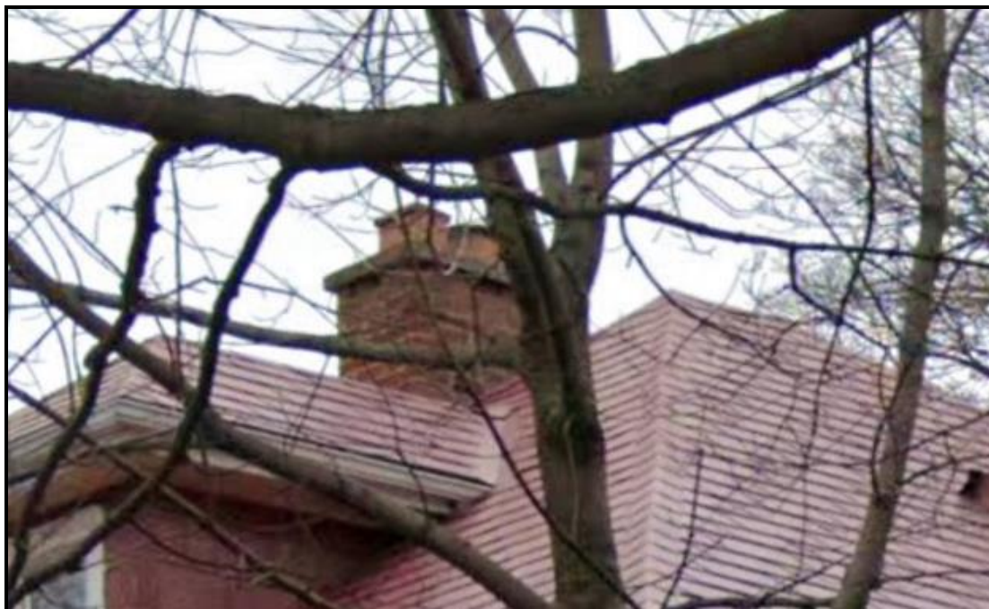
Close-up of the brick chimney, 2021. Source: Google
