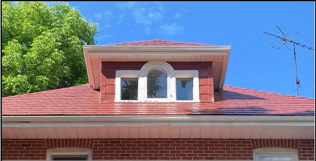
Palladian window in the front dormer, 2024. Source: Town of Oakville Planning Staff
