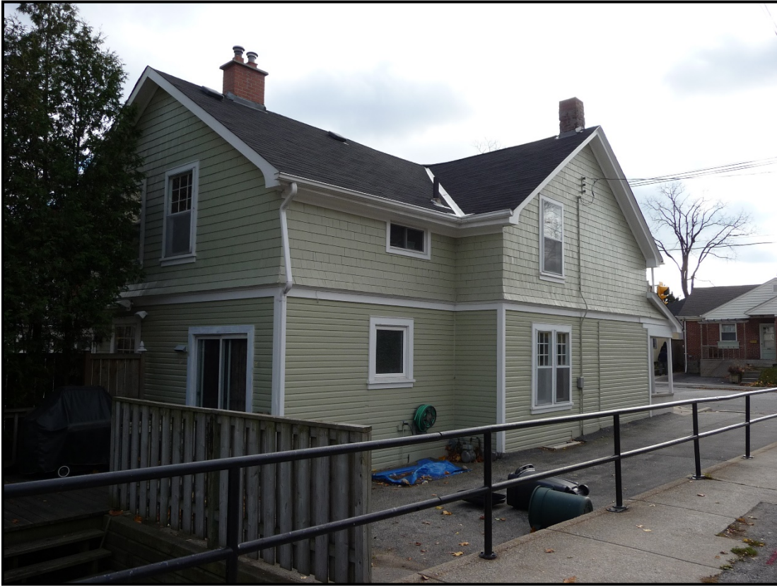
North elevation, showing the rear of the house from 137 Chisholm Street, 2024. Source: Town of Oakville Planning Staff
