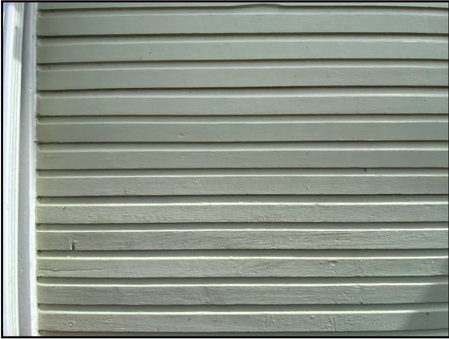
Close up of the wood horizontal siding, 2024. Source: Town of Oakville Planning Staff
