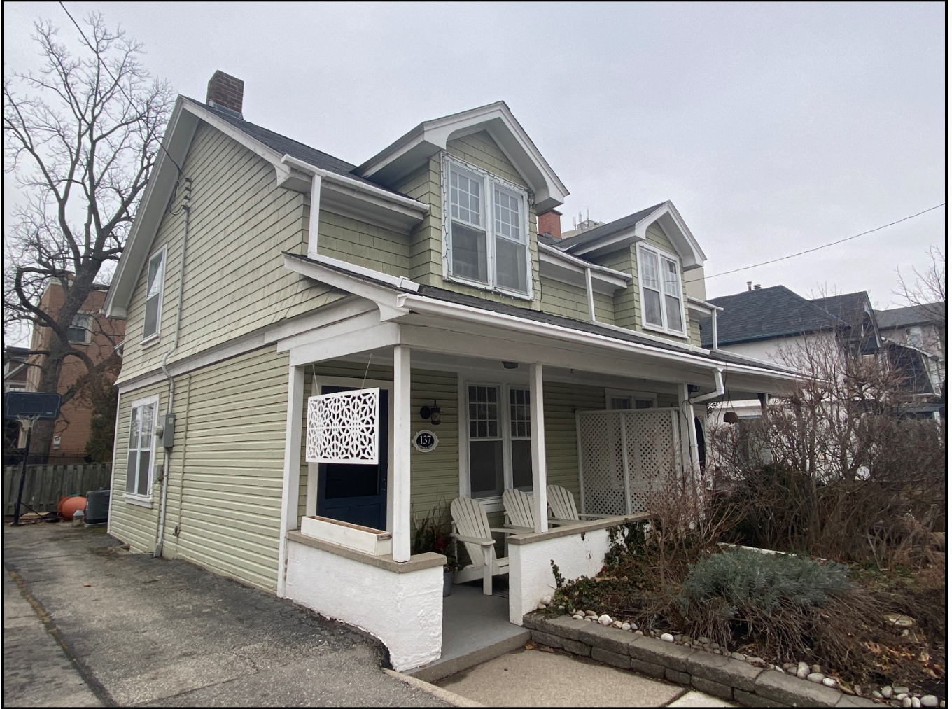
137 Chisholm Street, 2024. Source: Town of Oakville Planning Staff
