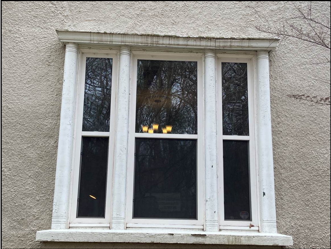
Close-up of the sash window with sidelights on the north elevation, which matches another one on the east elevation, 2024. Source: Town of Oakville Planning Staff
