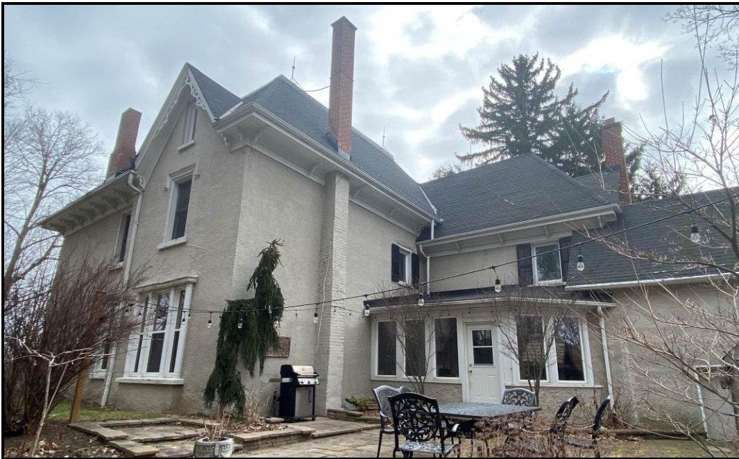
West and north elevations, 2024. Source: Town of Oakville Planning Staff
