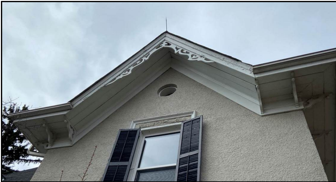
Photo showing the bargeboard and wooden soffit with decorative brackets, 2024. Source: Town of Oakville Planning Staff
