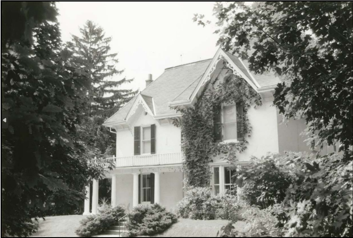
Undated Town photo showing the 2/2 style storm windows over the first storey windows. Source: Town of Oakville planning files
