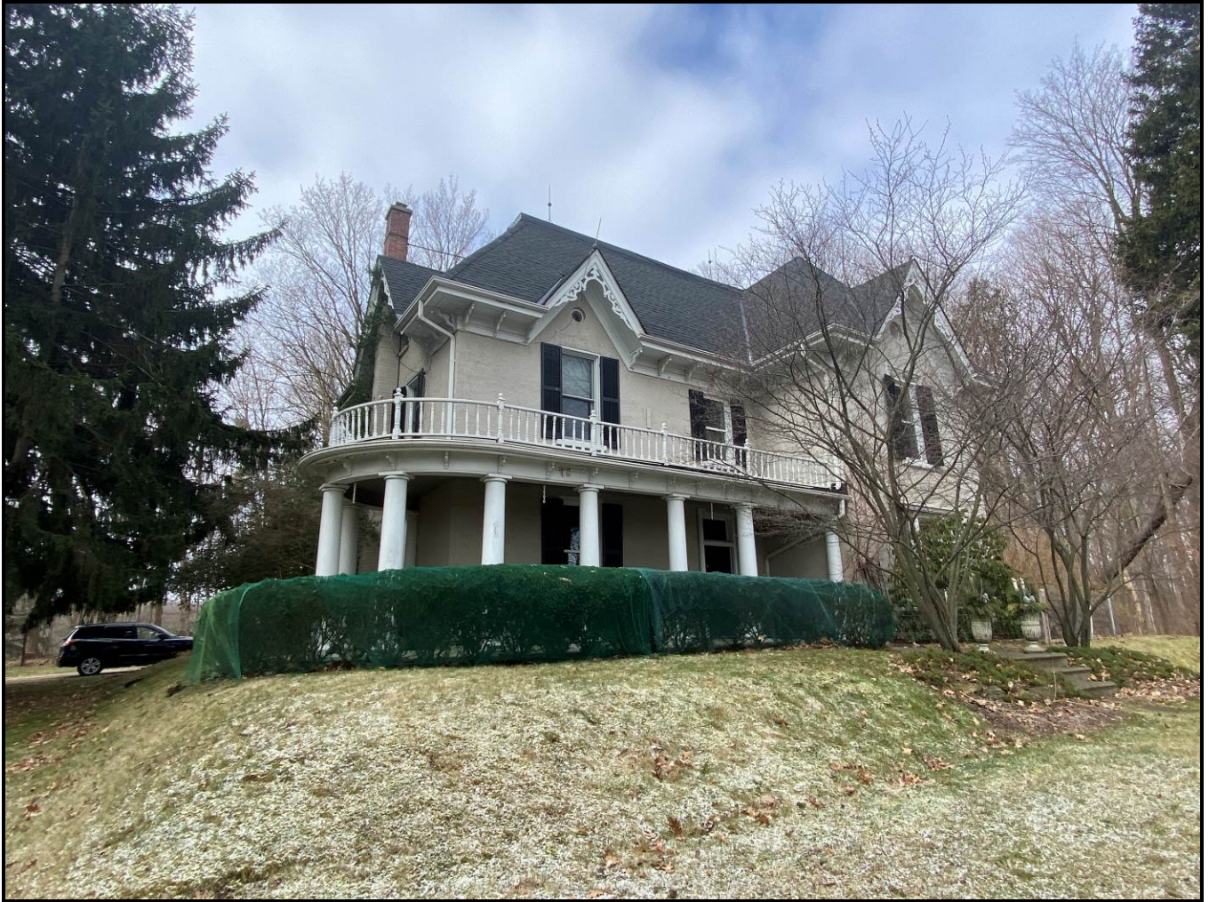
East elevation of 1242 Bronte Road, 2024. Source: Town of Oakville Planning Services Staff
