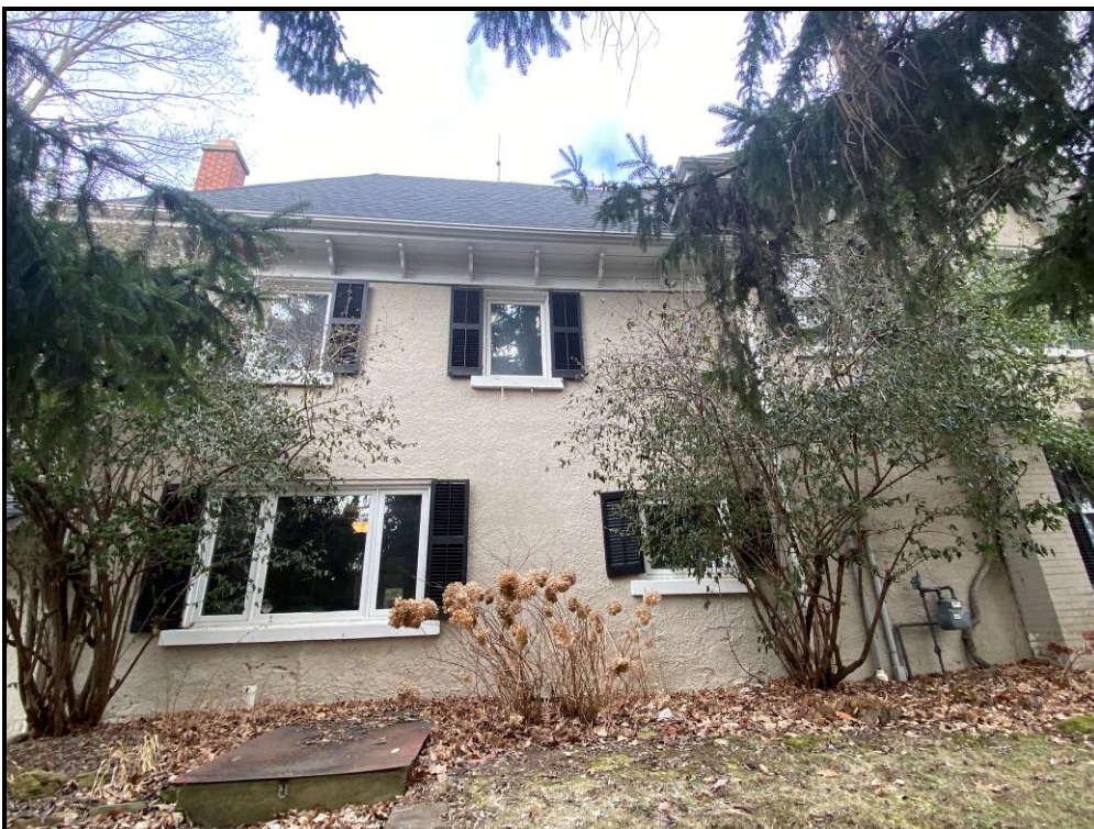
Modern windows have replaced some of the original windows on the south wall, 2024. Source: Town of Oakville Planning Staff
