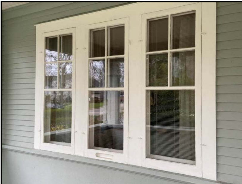
One set of the three windows on the first storey, showing the wooden trim and the historical multipaned windows and storm windows, 2024. Source: Town of Oakville Planning Staff
