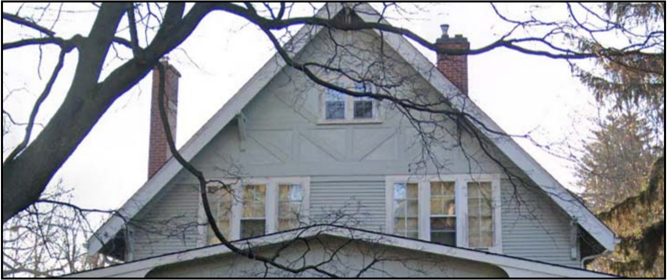
2021 photo showing the second storey and half storey windows, with multipaned sash windows. Source: Google
