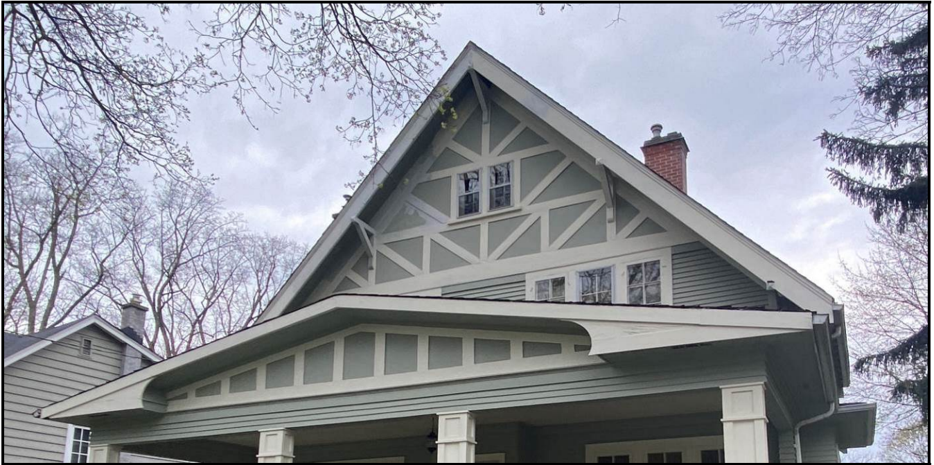
Close-up of the half-timbering on the front gable and porch. Directly underneath the half-timbering the horizontal wood siding starts again, 2024. Source: Town of Oakville Planning Staff
