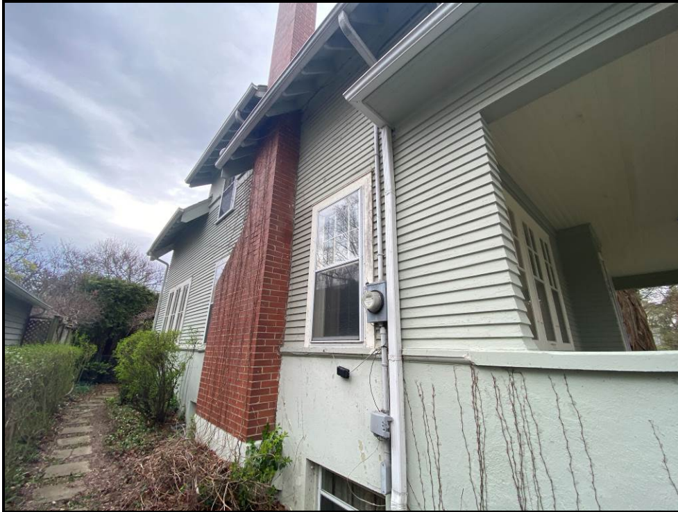
Chimney on east elevation, 2024. Source: Town of Oakville Planning Staff
