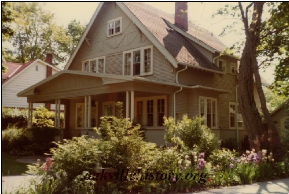
Replacement pillars as separated columns, 1980s. Source: Oakville Historical Society
