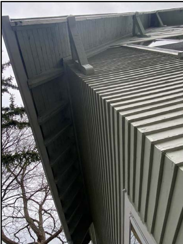
Close-up of the wooden soffit, projecting eaves, and large brackets on the roof trim, 2024. Source: Town of Oakville Planning Staff
