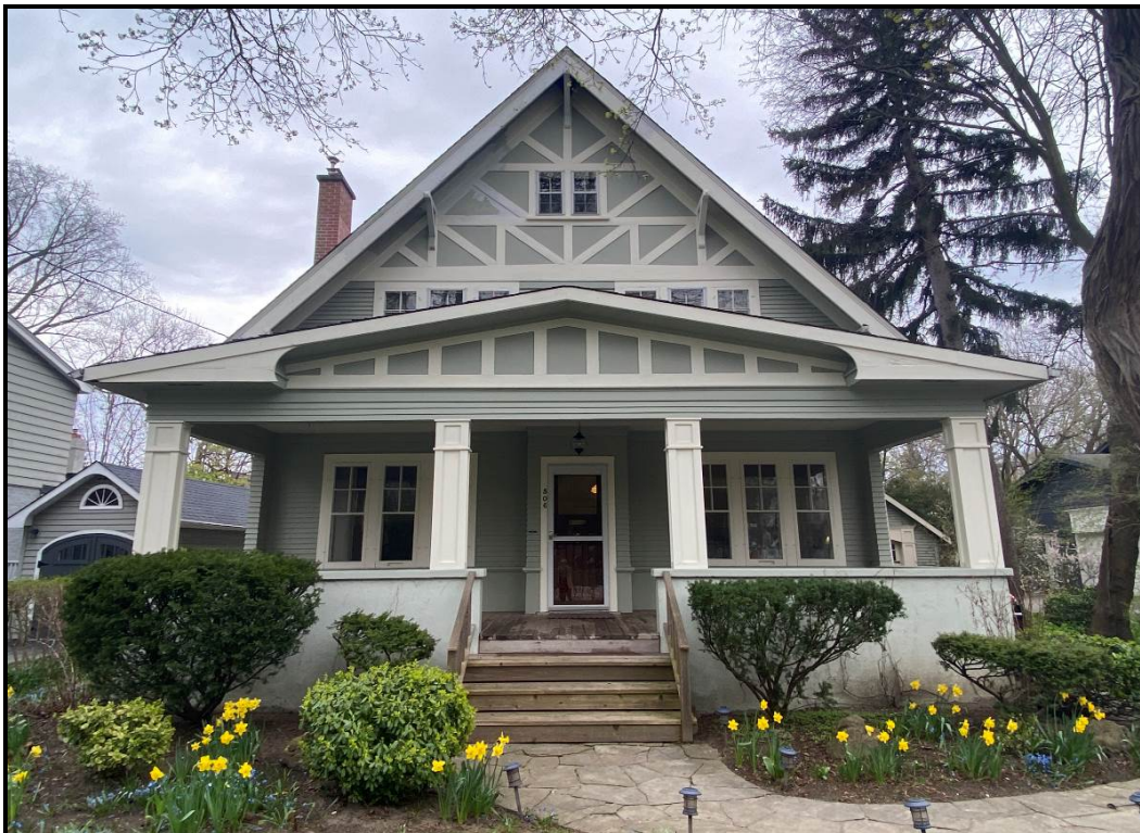
Front and east elevations showing porch roof overhang with wide eaves, and the front gable of the main house, 2024. Source: Town of Oakville Planning Staff
