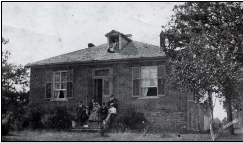
The Nisbet and later Bacon family home, known as "The Manse", built in the 1850s. It was one of the earliest structures in the large historical Lot 11. Samuel Bacon developed the area around it, with Carson developing lands to the east. Source: Oakville Historical Society
