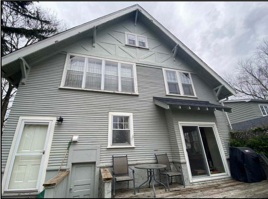
South (rear) fenestration, showing multipaned sash windows of 4/1 and 6/1, 2024. Source: Town of Oakville Planning Staff
