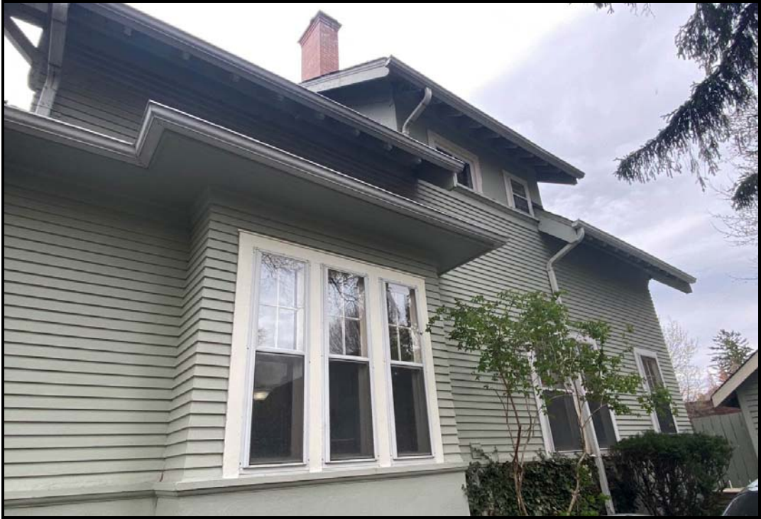
Shed dormer and unique porch roof overhang that wraps around both east and west elevations, with a projecting window, 2024. Source: Town of Oakville Planning Staff
