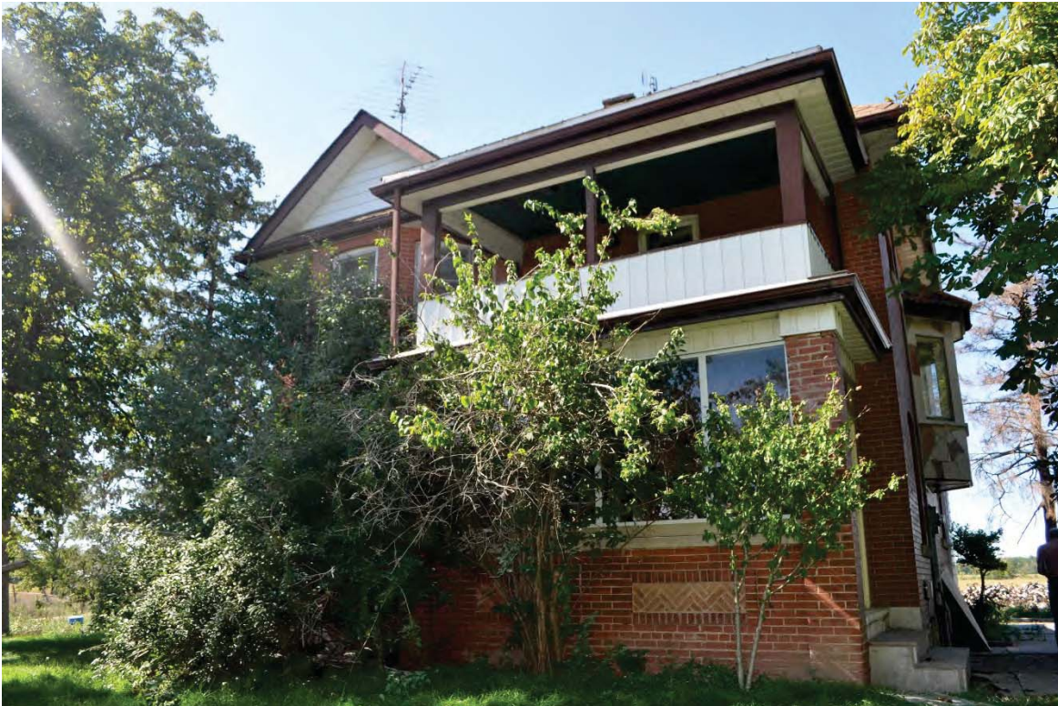
Figure 8: 3367 Dundas Street West, front facade (CU 2016).
