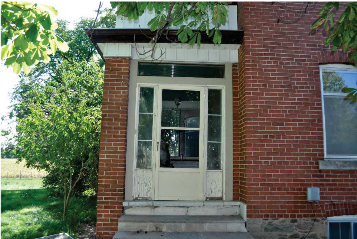
Figure 11: 3367 Dundas Street West, front porch and foundations, east façade (CU 2016).
