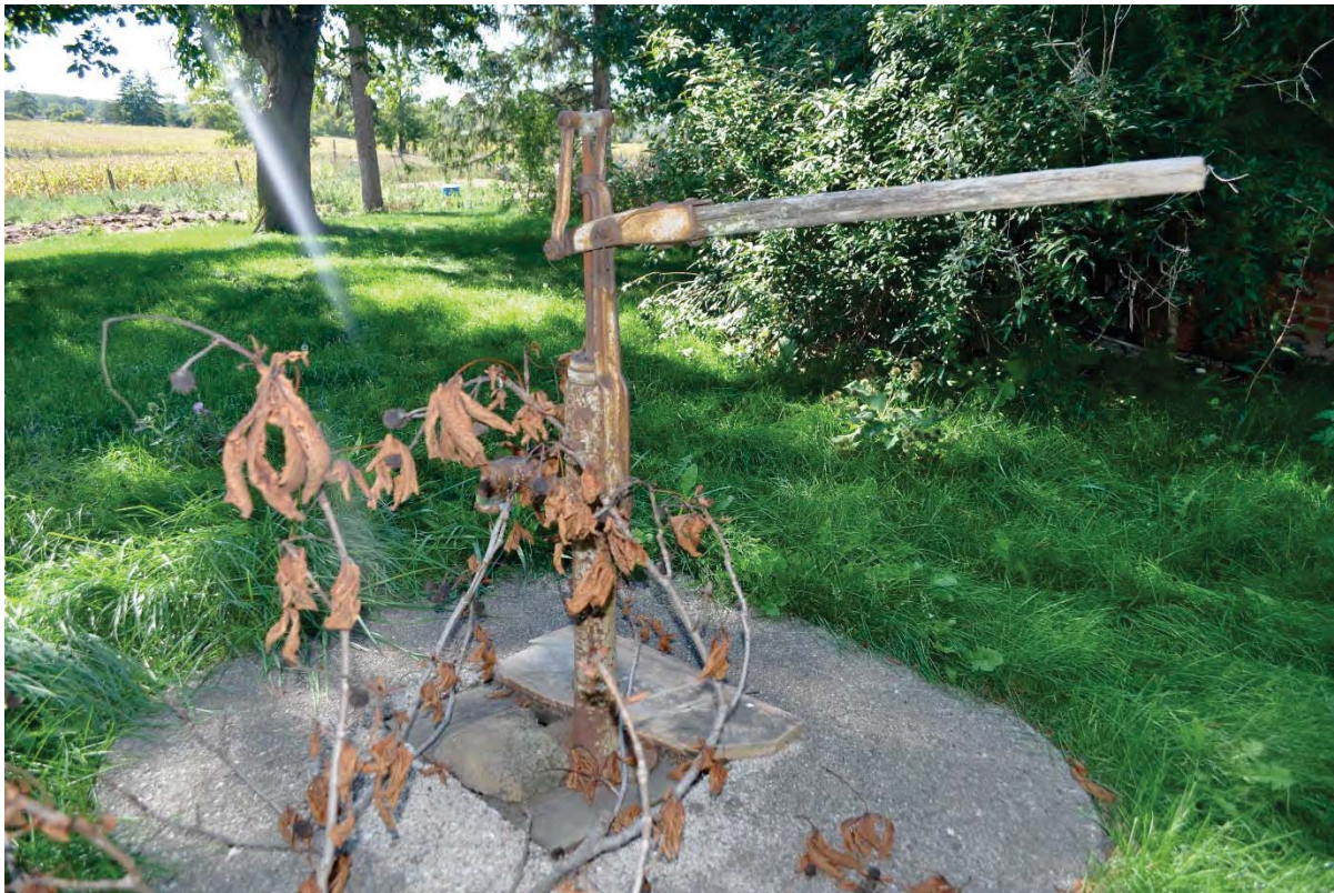
Figure 16: Well pump south of residence (CU 2016).
