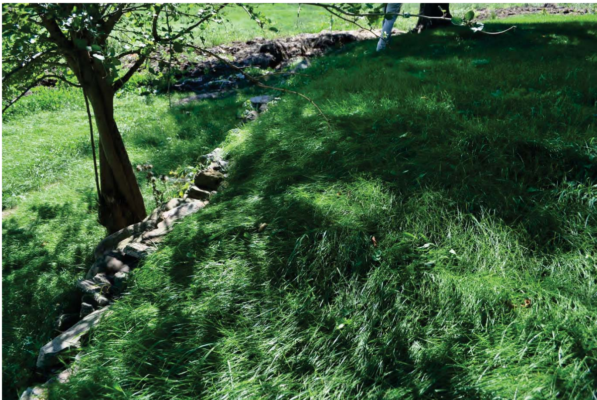
Figure 17: Retaining wall (CU 2016).
