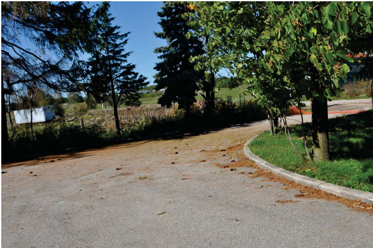
Figure 14: Driveway detail, east of residence (CU 2016).
