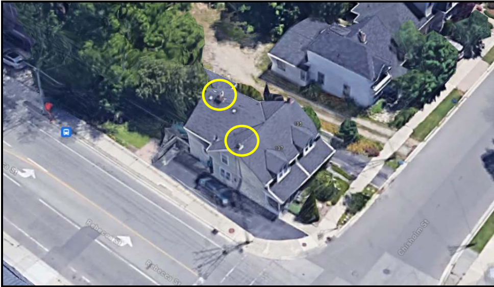
Chimneys from the aerial. Source: Google
