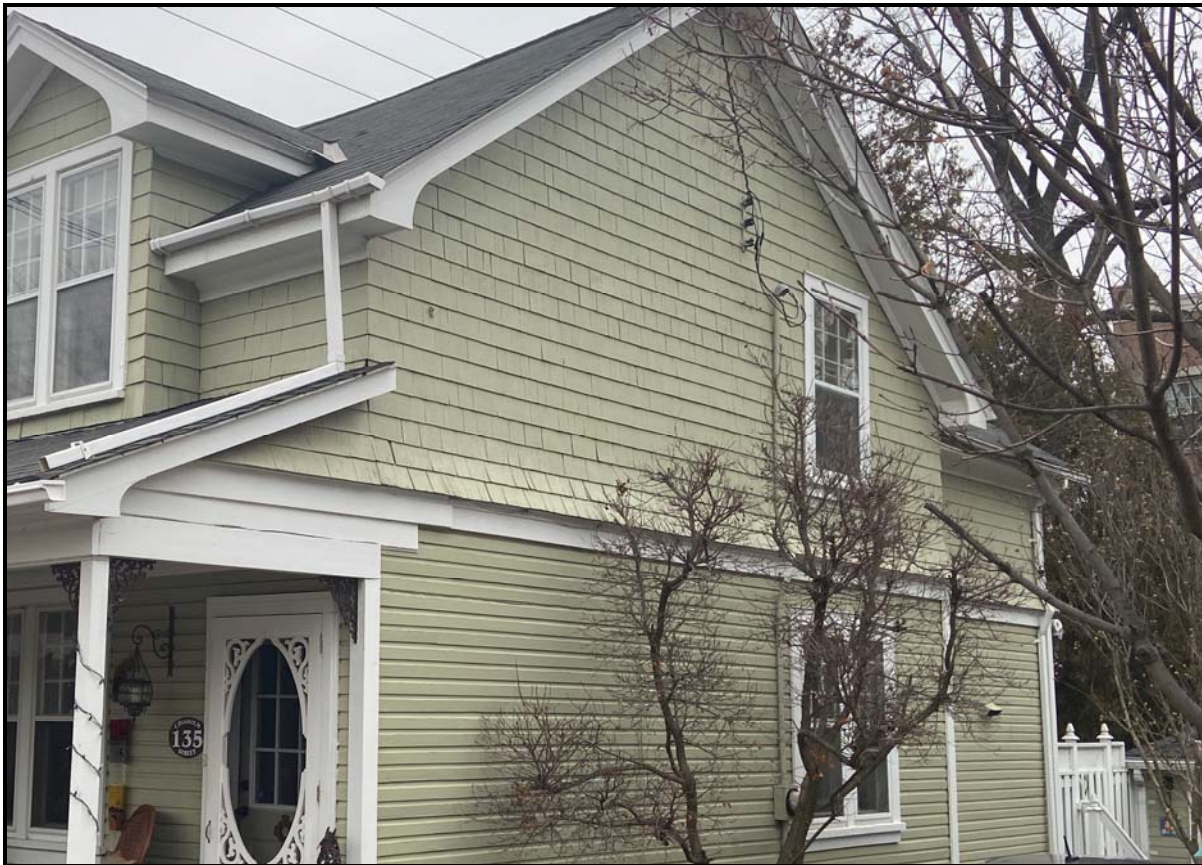
Siding on 135 Chisholm Street, showing the shingles and horizontal siding, 2024. Source: Town of Oakville Planning Staff
