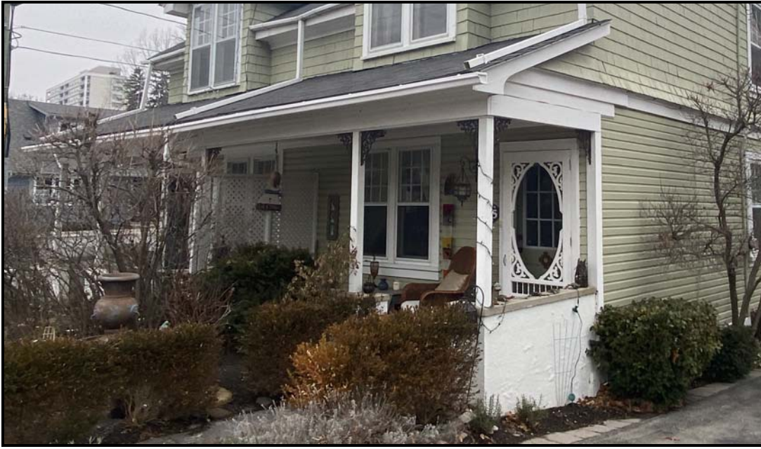
Front porch with simple square columns and a stucco knee wall at 135 Chisholm Street, 2024. Source: Town of Oakville Planning Staff
