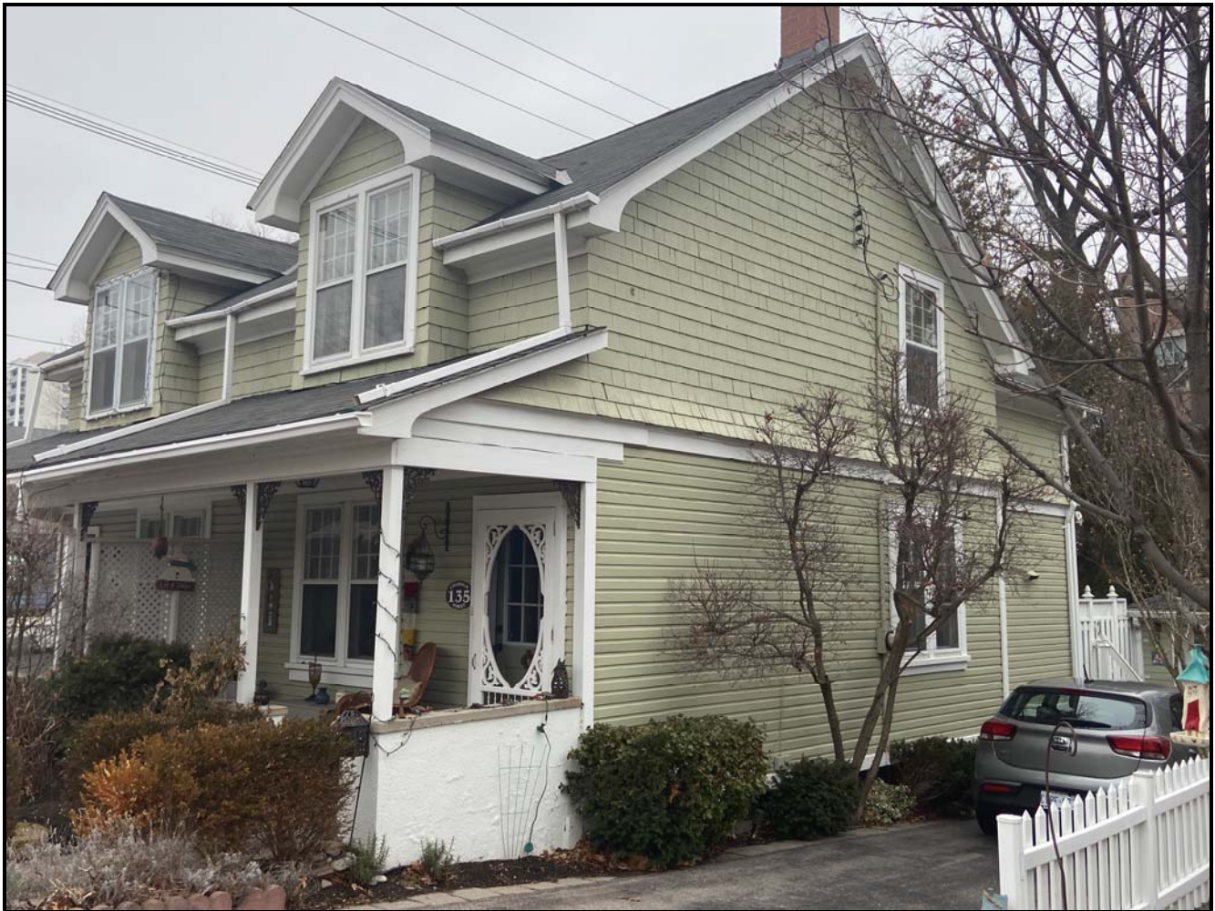
View of the west elevation (front) and south elevation of 135 Chisholm Street, 2024. Source: Town of Oakville Planning Staff
