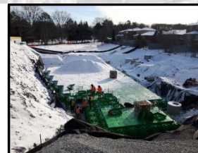
OPEN BOTTOM FACILITY
