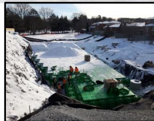
OPEN BOTTOM FACILITY
