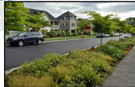
Alt 3B: Local (minor) Ditch System Improvements with LID/Green Infrastructure enhancement (Bioswale)
