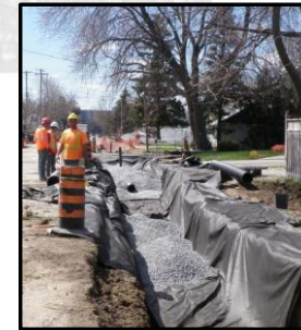
Alt 4B: LID/ Green Infrastructure enhancement (perforated pipe) to existing storm sewer upgrades and new storm sewers)
