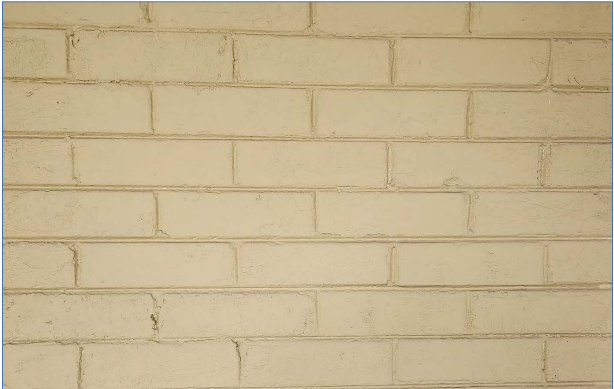
Photo 9: View southeast showing a section of the painted stretcher bond brick
