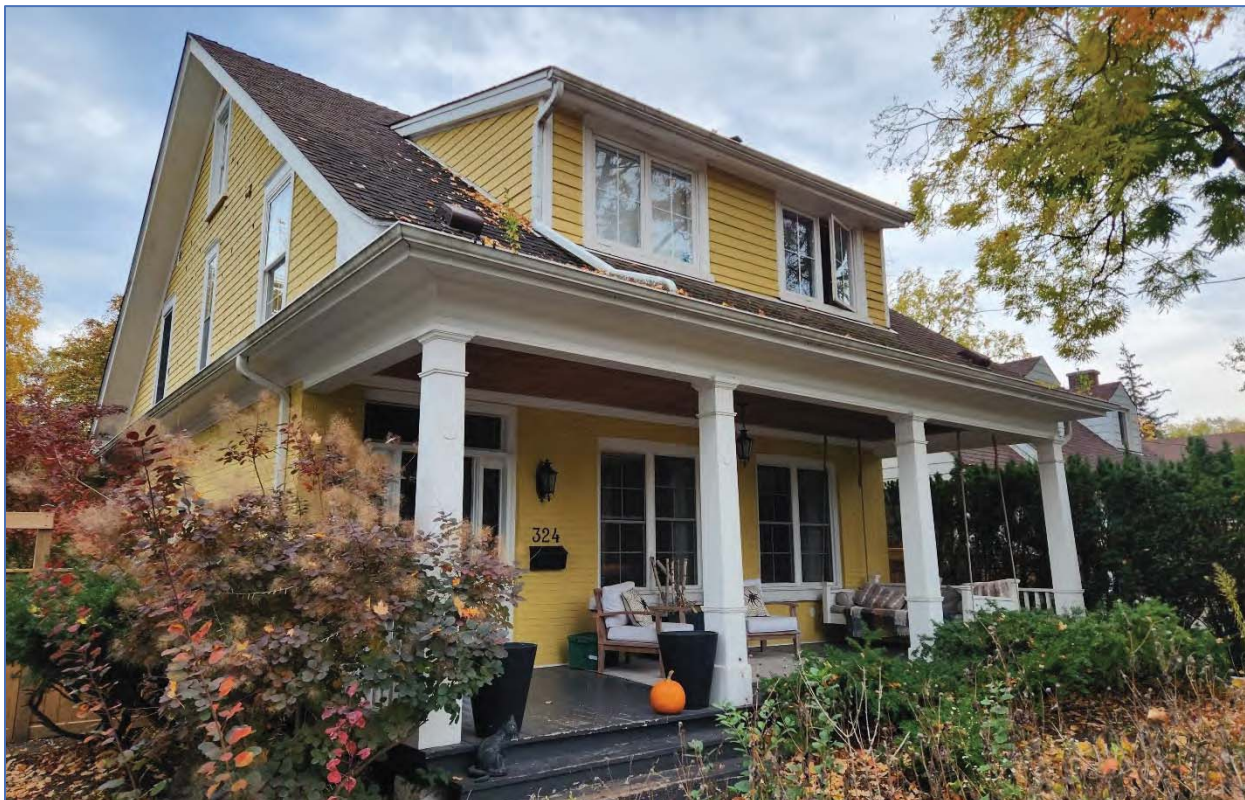
Photo 13: View south showing the roof profile
