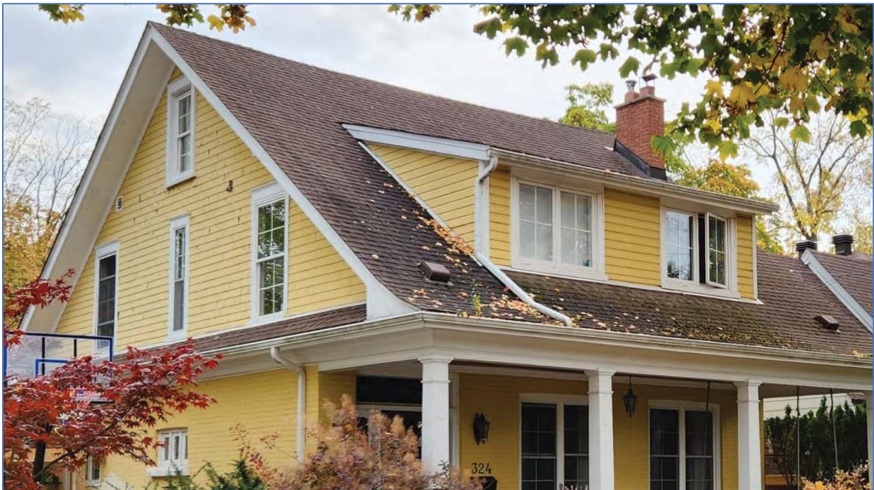
Photo 19: View south showing gable end and dormer windows
