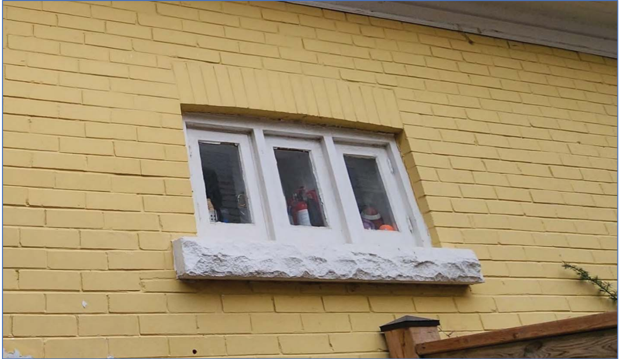
Photo 16: View southwest showing the three-sash window on the northeast elevation
