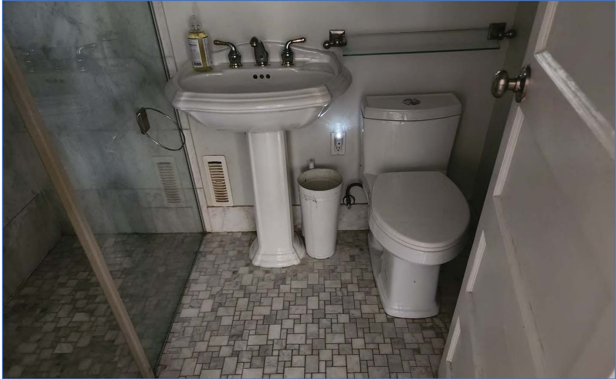
Photo 24: View northwest showing the first storey bathroom
