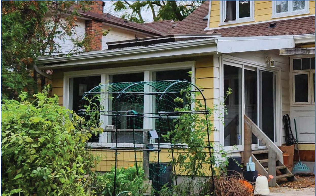
Photo 18: View northwest showing the rear wing addition
