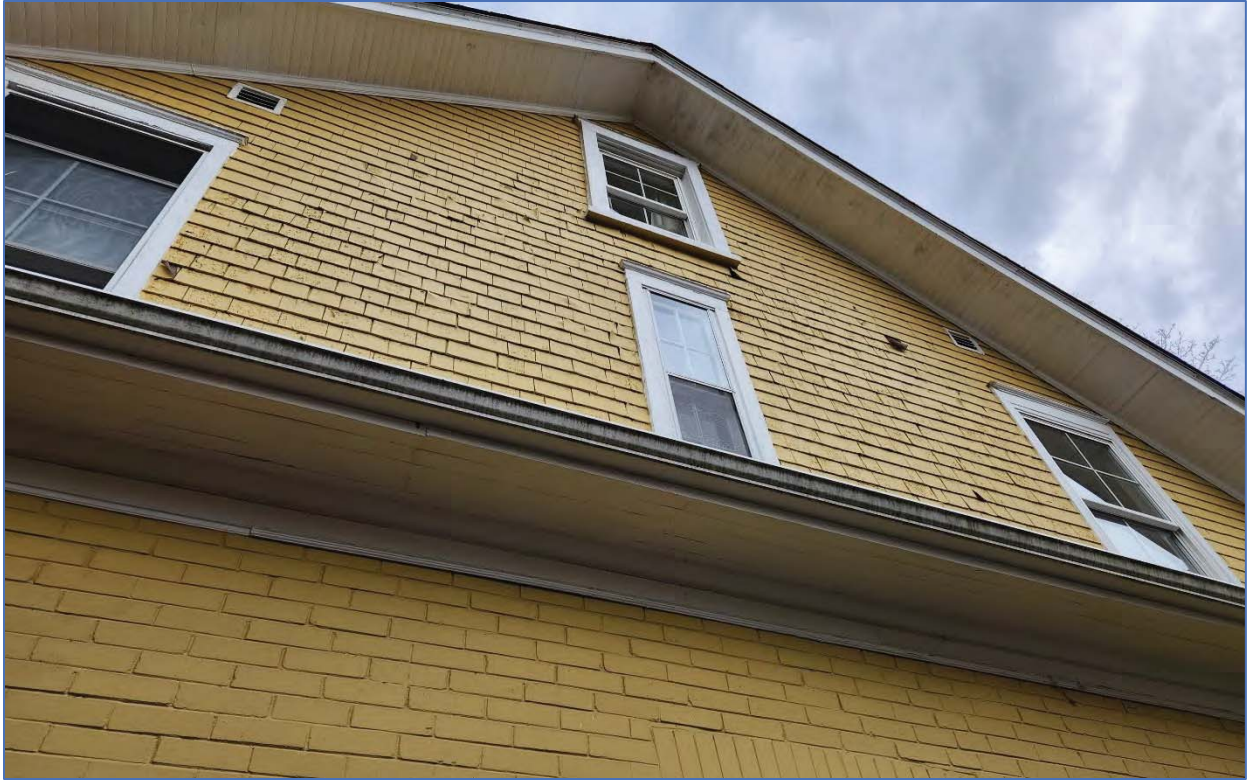
Photo 10: View southwest showing cedar shakes in the northeast gable end
