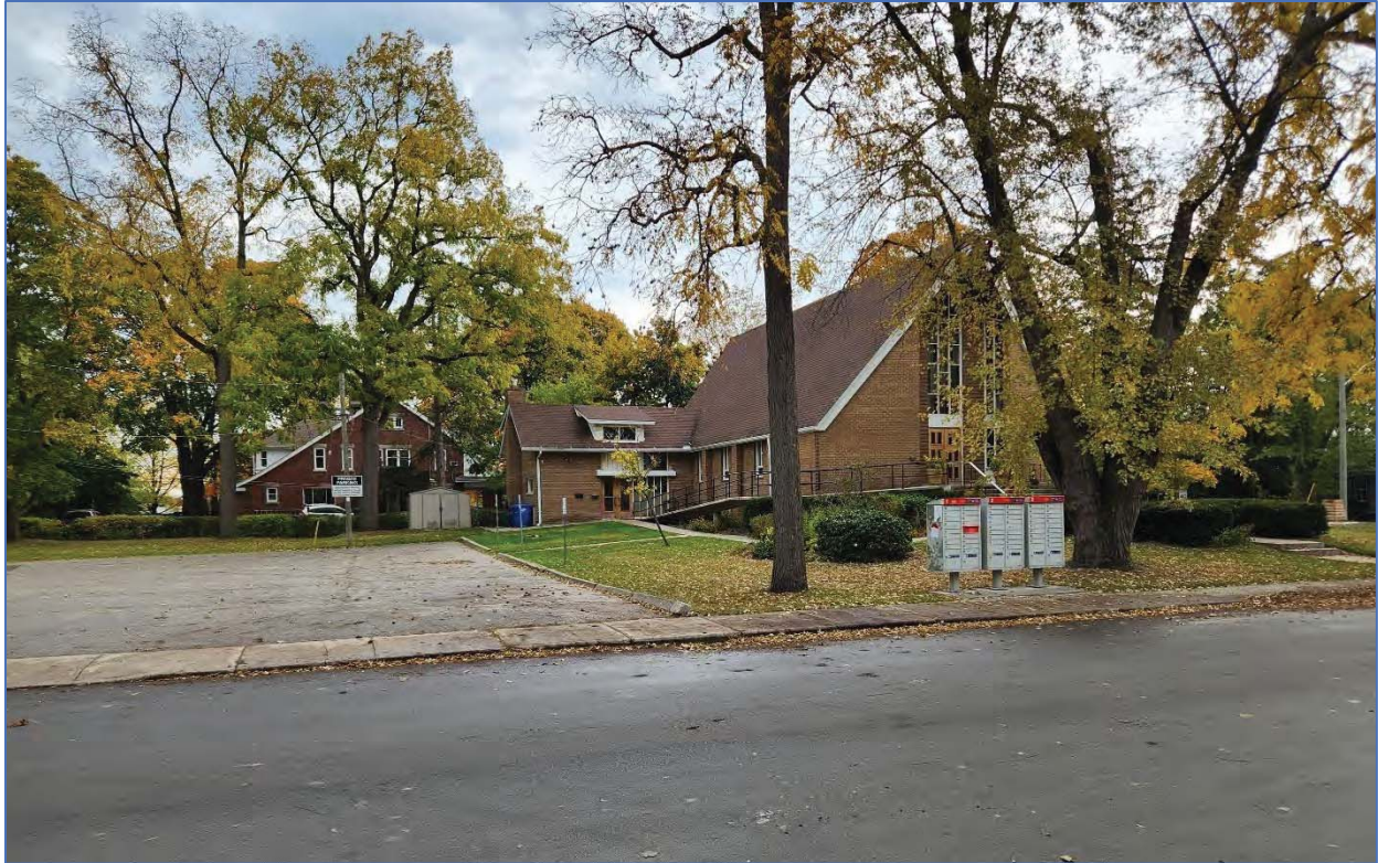
Photo 5: View southeast of the church at 318 Spruce Street
