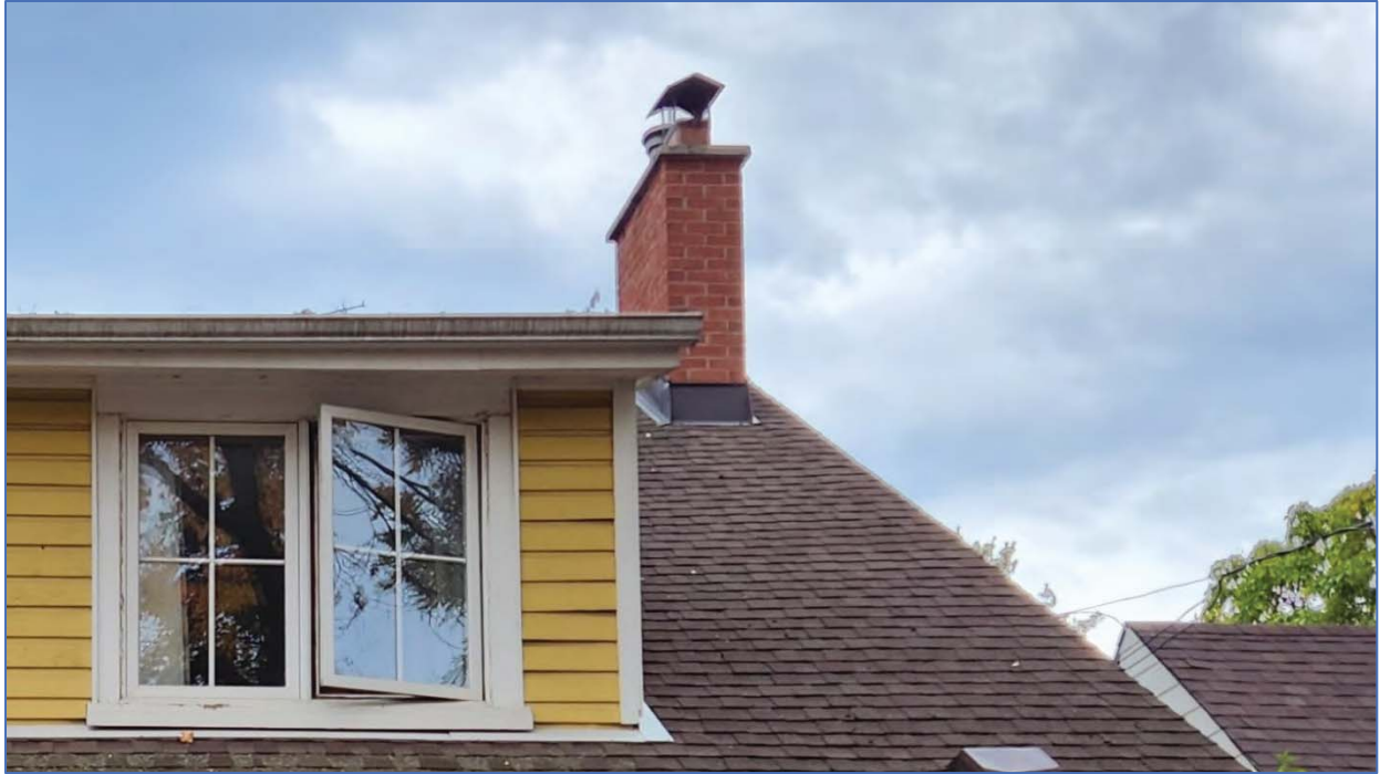
Photo 14: View southeast showing the chimney
