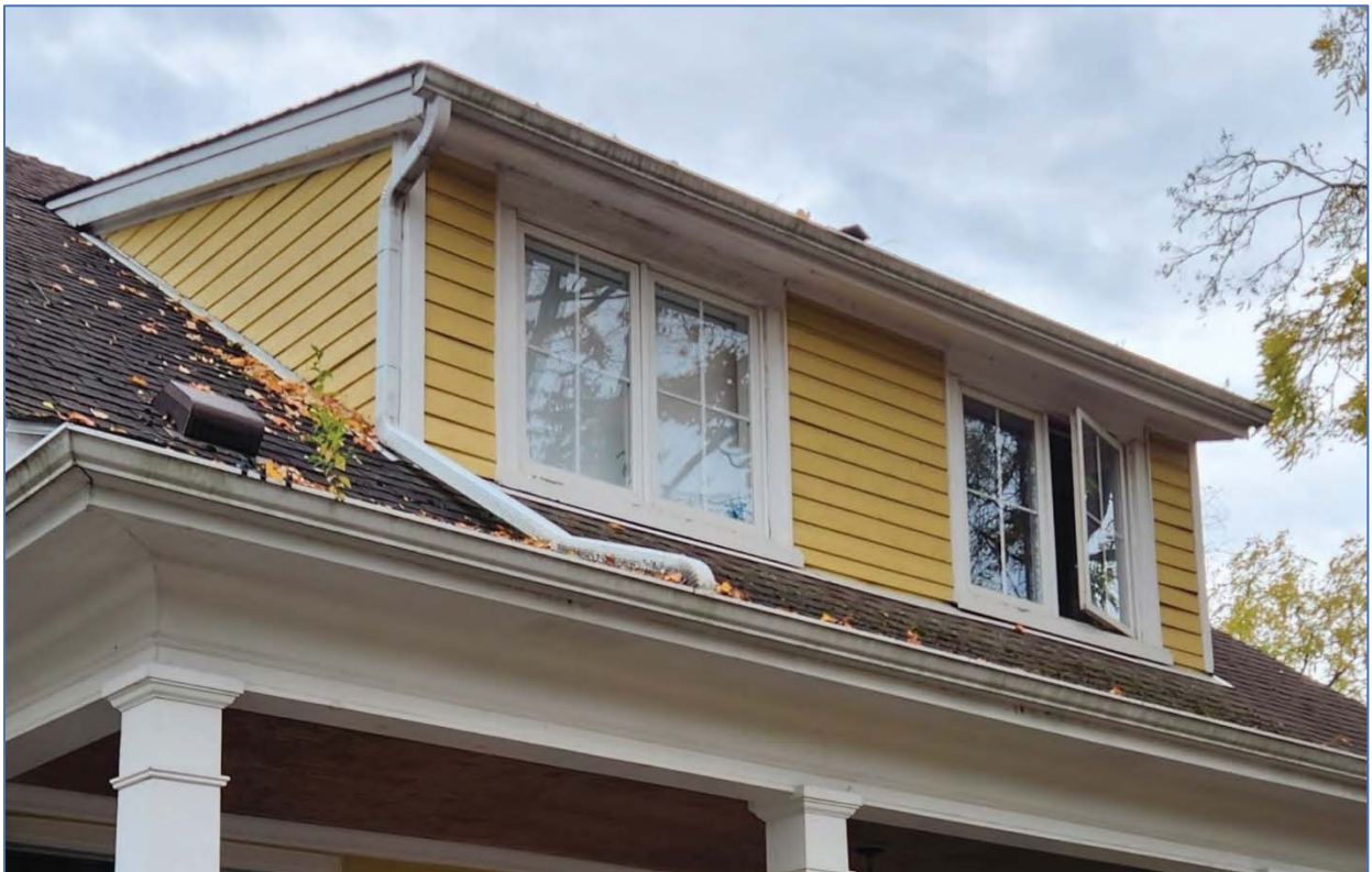
Photo 11: View south showing the clapboard siding on the northwest dormer
