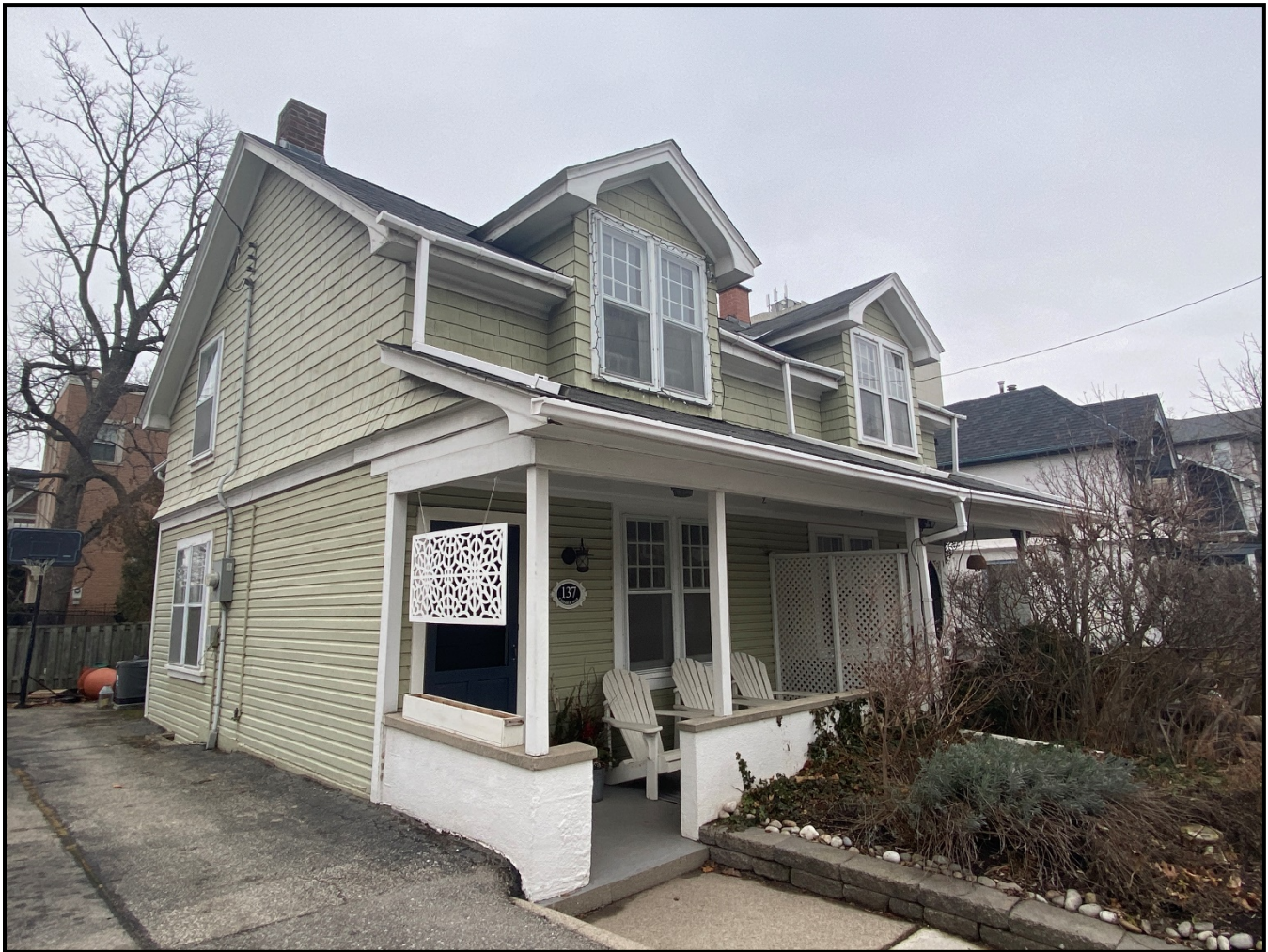
View of the west elevation (front) and north elevation of 137 Chisholm Street, 2024. Source: Town of Oakville Planning Staff
