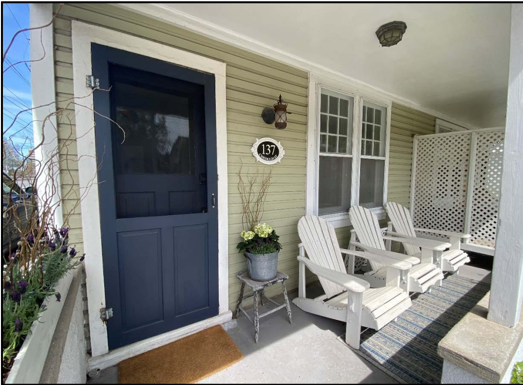
The front door and front porch of 137 Chisholm Street, 2024. Source: Town of Oakville Planning Staff
